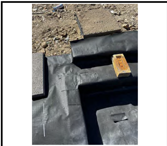
CQA photographic evidence of the JUTA GP1 Gas Barrier line out installation within Plots 592 & 593.
