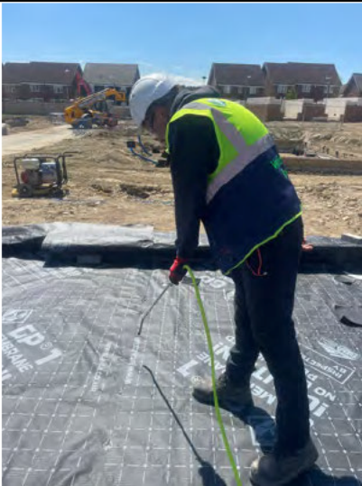
Air lance test on a welded lap.
