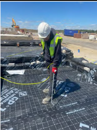
Air lance test on a welded lap.
