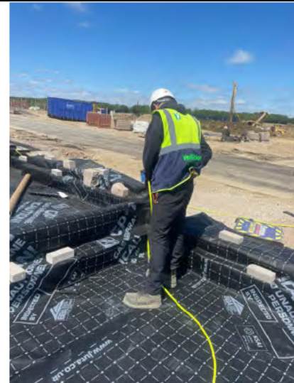
Air lance test on a corner.
