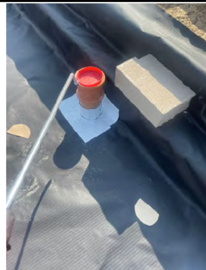
Air lance test on a pipe penetration.
