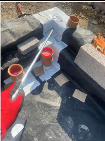
Air lance test on a pipe penetration.
