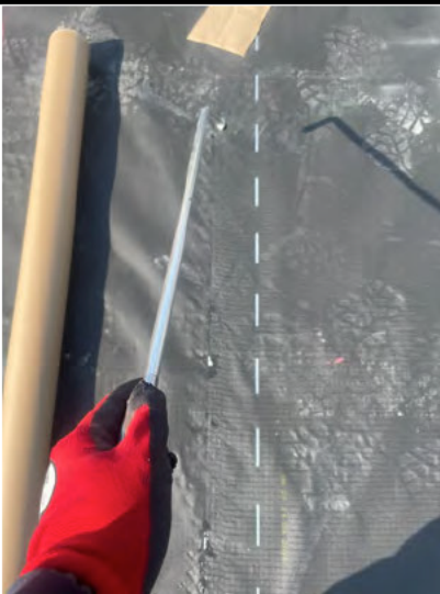
Air lance test on a welded lap.
