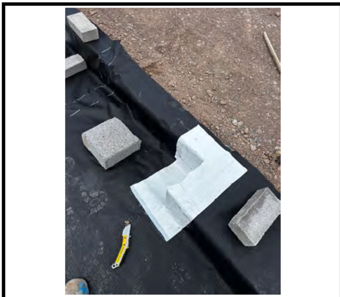
Typical corner detailing.
