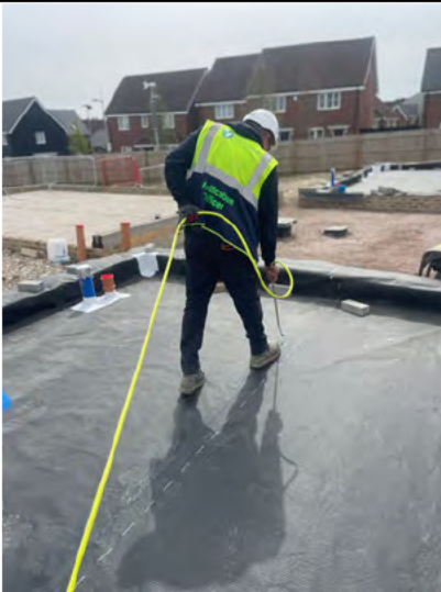
Air lance test on a welded lap.
