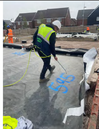
Air lance test on a welded lap.
