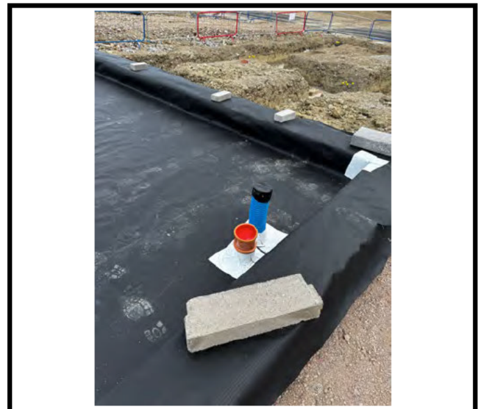
Typical pipe penetration detailing.
