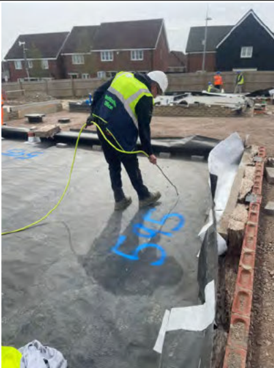
Air lance test on a welded lap.
