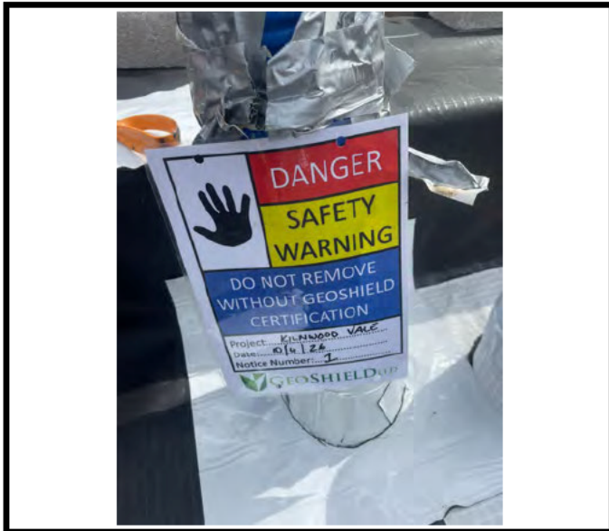
GeoShield safety warning notices placed around details to be sealed internally at a later date.
