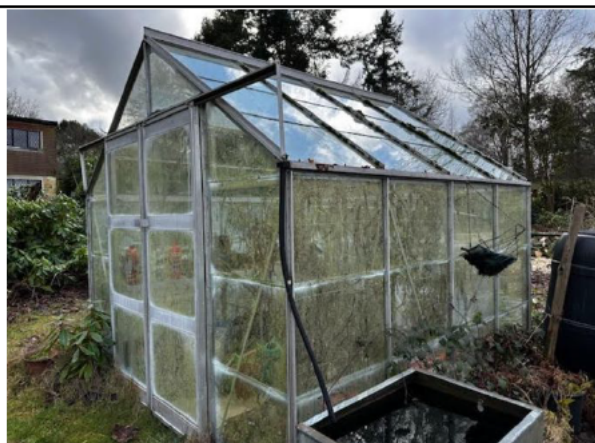
Photograph 17 – The glass greenhouse (B3) will be demolished as part of the proposed works.
