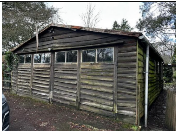
Photograph 15 – The wooden garage/sunroom detached building (B2) on site proposed to be demolished.
