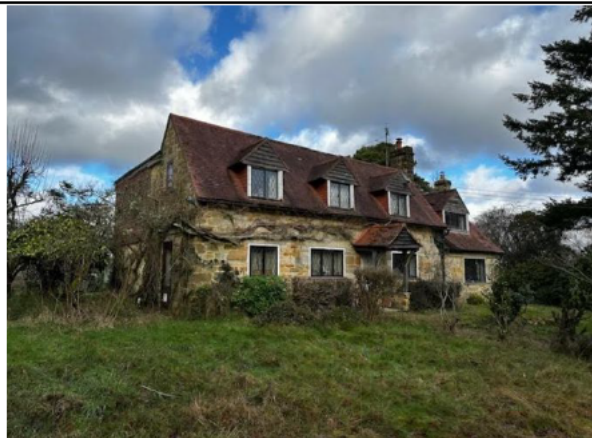
Photograph 3 – Part of the southwest elevation and the southeast elevation of the existing dwelling on site.
