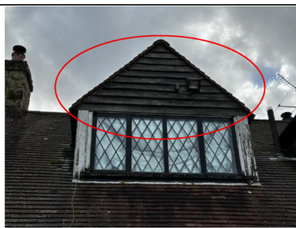
Photograph 8 – The dormer windows on the southeast and southwest elevations were covered with wooden weather boarding. The weatherboarding was well weathered and large gaps were not visible from the ground level assessment.
