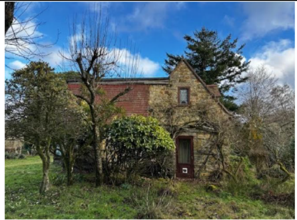
Photograph 2 – The southwest elevation of the existing dwelling on site.
