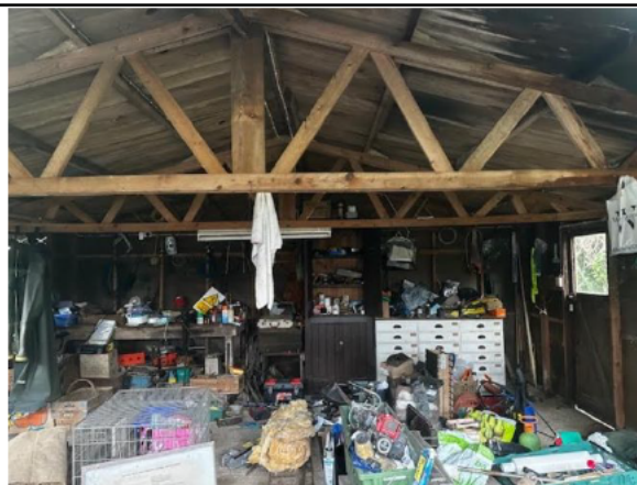
Photograph 16 – The internal view of the wooden garage/sunroom detached building (B2) with no void present.
