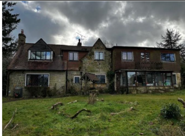
Photograph 1 – The northwest elevation of the existing dwelling (B1) on site proposed to be demolished.
