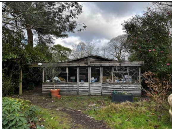
Photograph 14 – The wooden garage/sunroom detached building (B2) on site proposed to be demolished.
