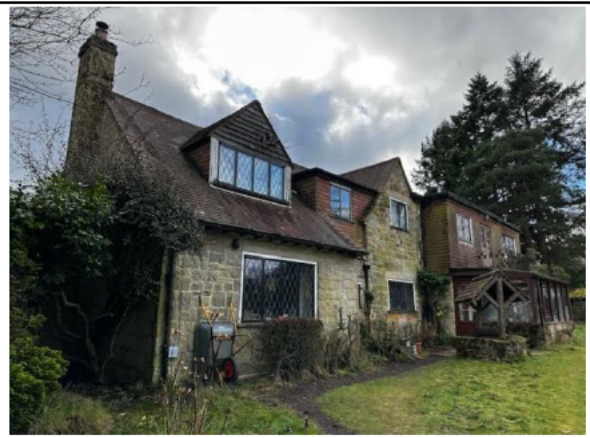
Photograph 4 – Part of the northeast elevation and part of the northwest elevation of the existing dwelling on site.
