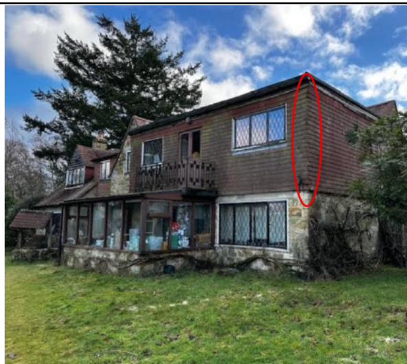
Photograph 5 – A large area of the northwest and southwest elevations were tile hung with concrete hanging tiles.
