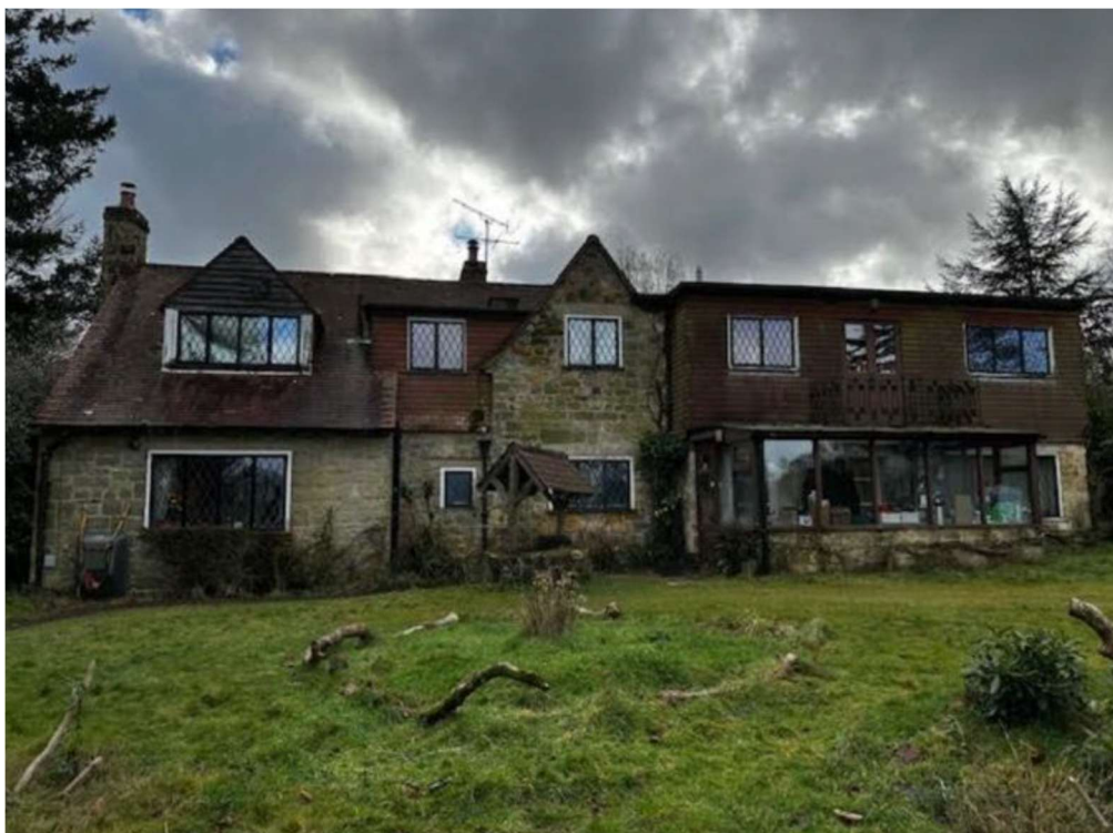
Figure 10: View of the building to be demolished
