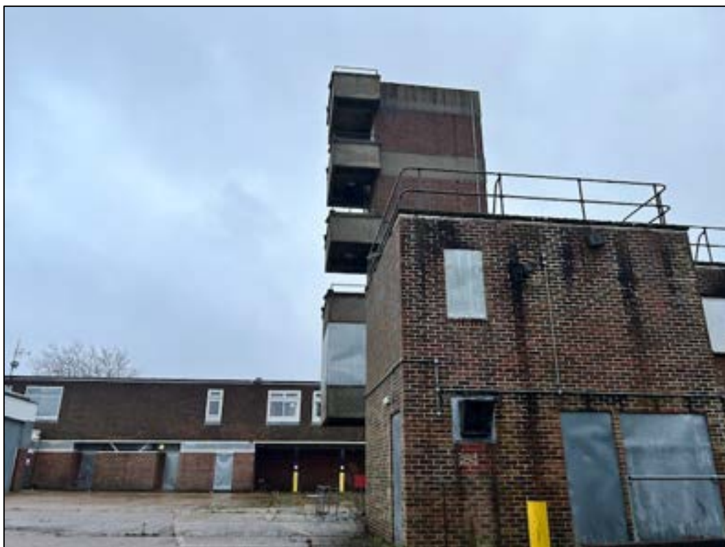
Training building and tower in west of site
