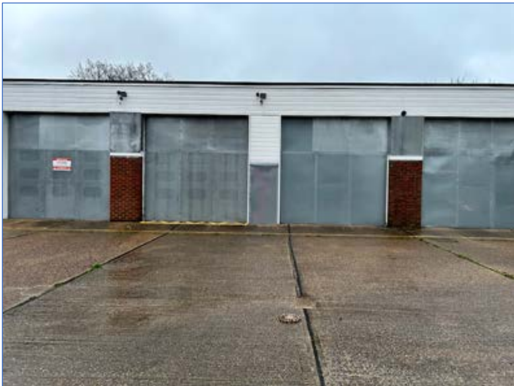
Rear of main building looking north east
