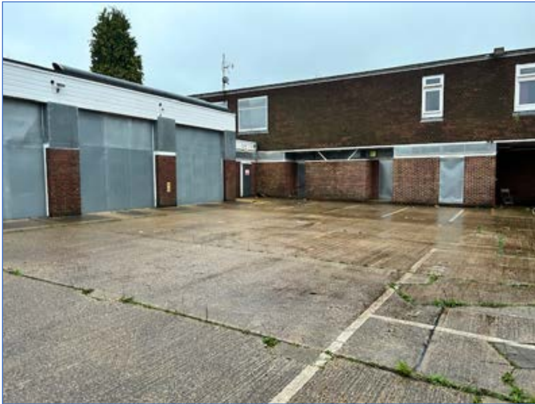
Rear of main building looking east
