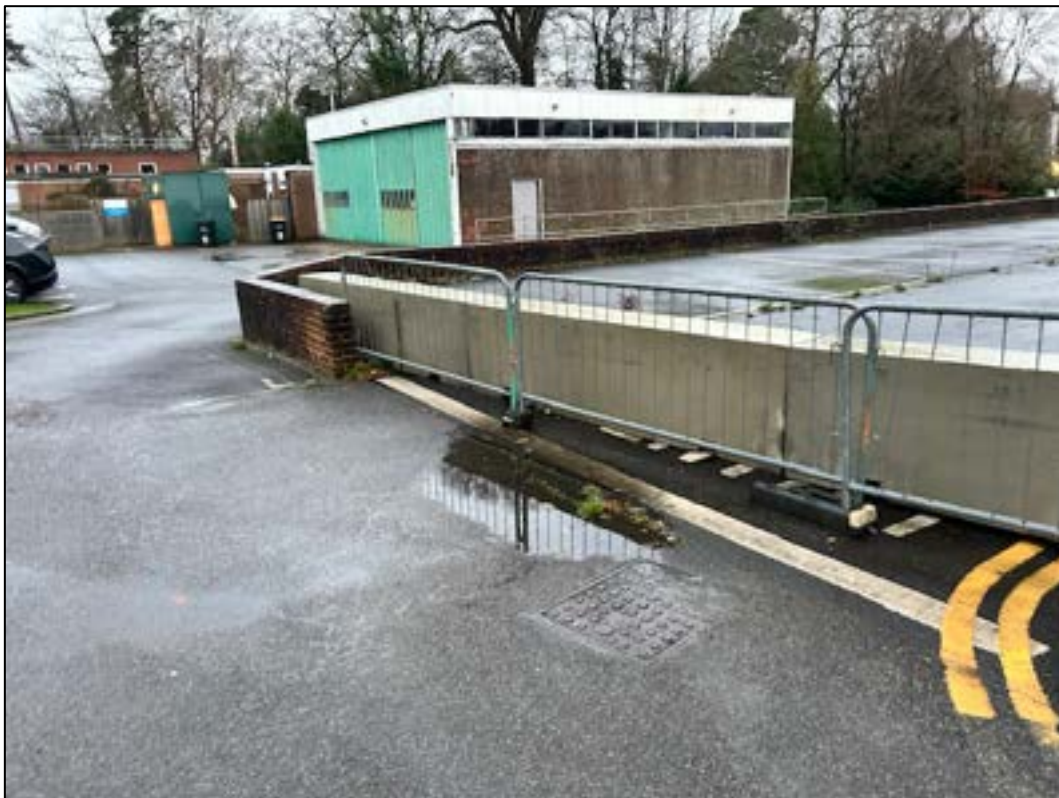
Access at southern corner of site
