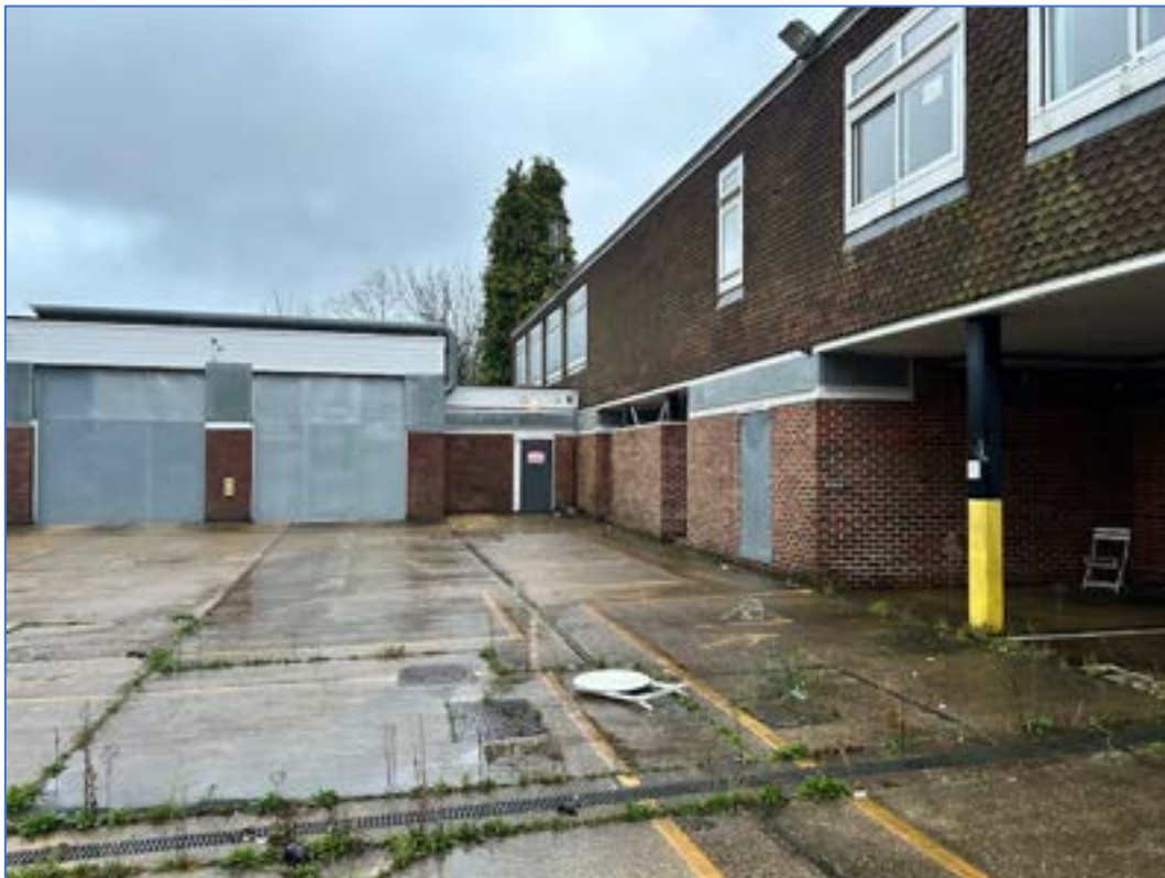
Rear of main building looking north east
