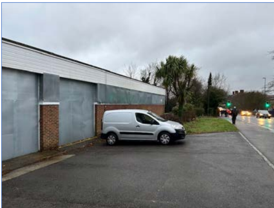
View north west along site frontage showing appliance entrance
