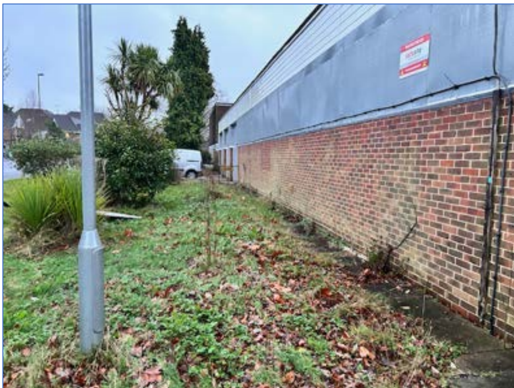
View south east along site frontage and Hurst Road
