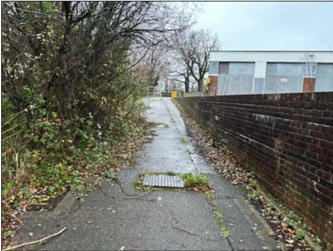
View north east along site boundary showing retaining wall
