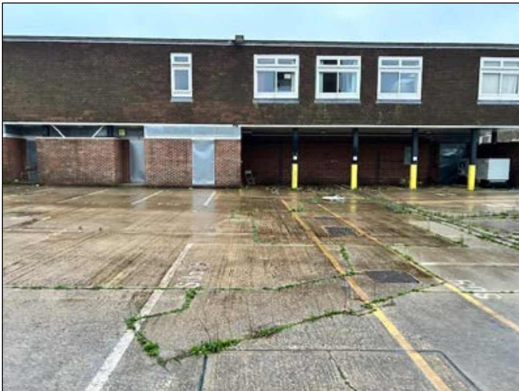
Rear of main building looking south east showing car ports
