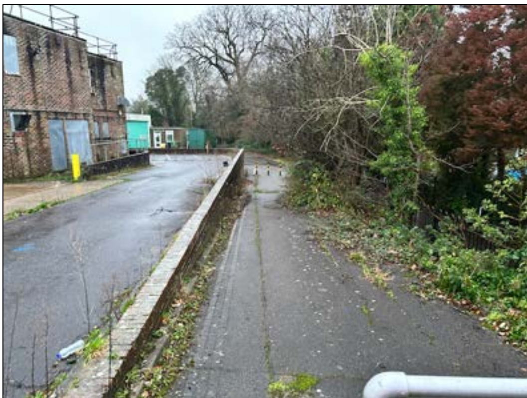
View south west showing retaining wall on north western boundary
