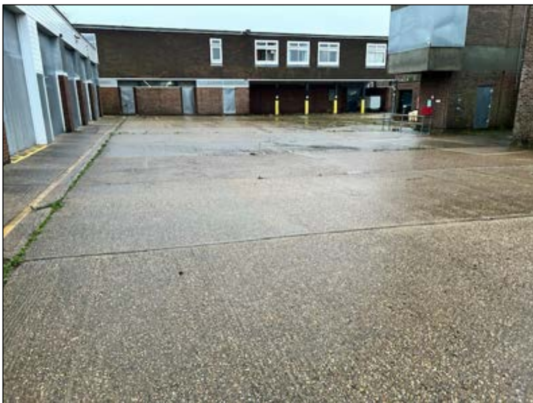
View of rear yard looking south east
