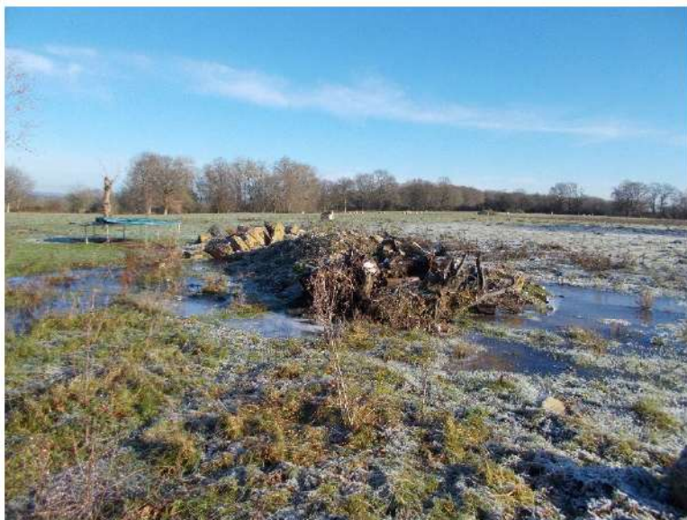
Photograph 5: Pile of brash (cut / felled wood), mixed soil and building rubble, large section of concrete slab / rubble.
