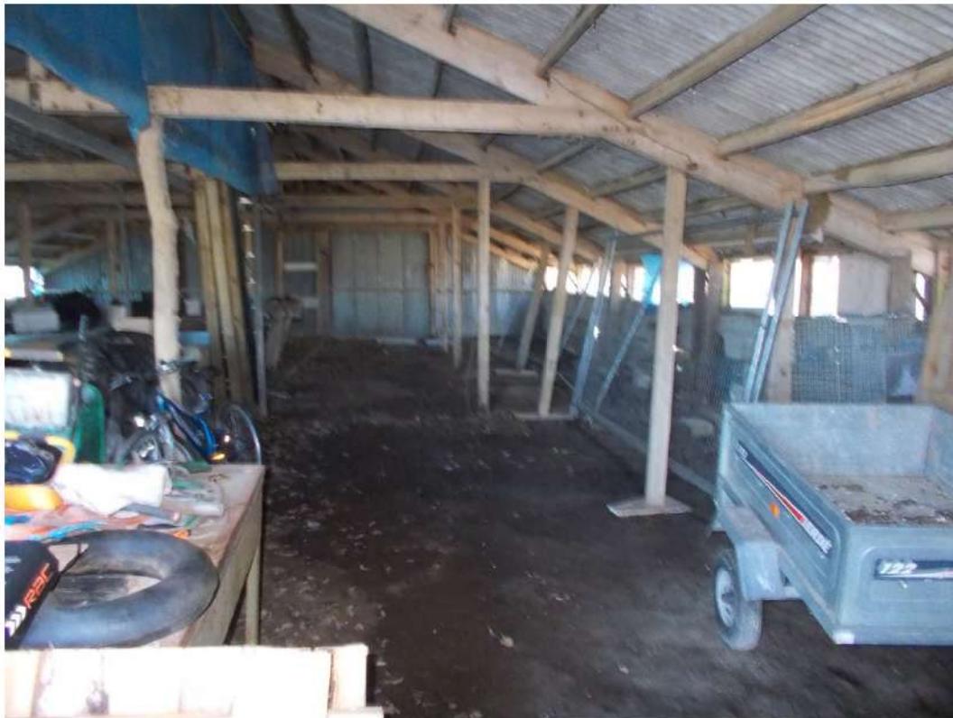
Photograph 8: Northern section of the shed with compressed dirt floor.
