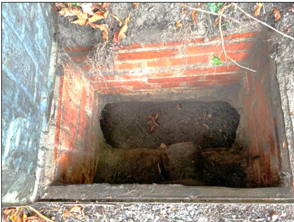
Figure 2.4 – Surface Water Manhole with Incoming Highways Drainage
