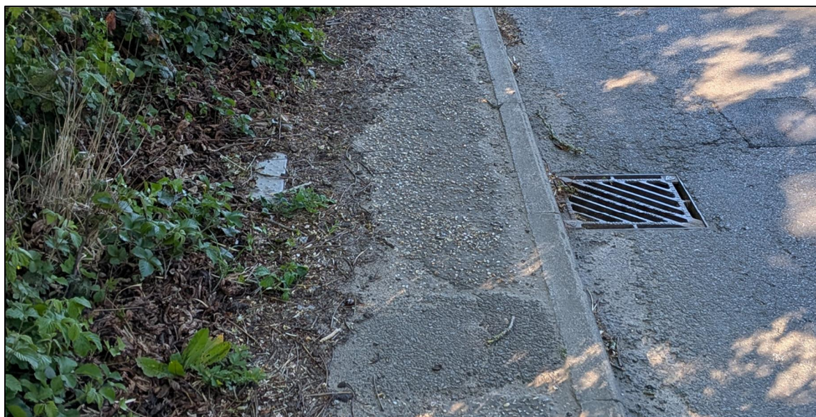
Figure 2.5 – Proximity between Highway Gully and Manhole
