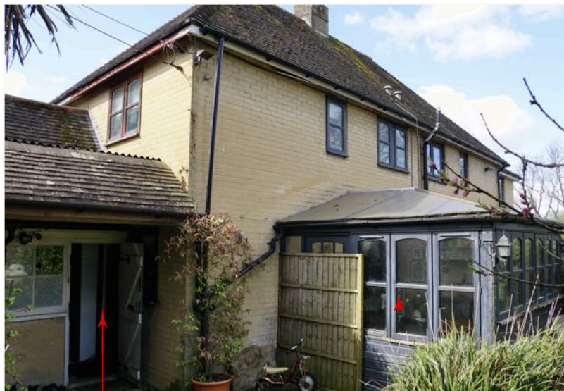
EXISTING ENTRANCE & CONSERVATORY
