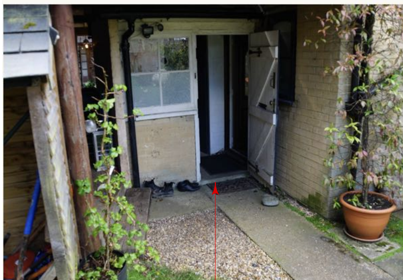
EXISTING PORCH ENTRANCE
