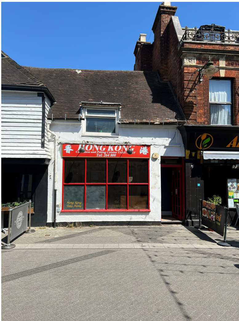
25 East Street - front view
