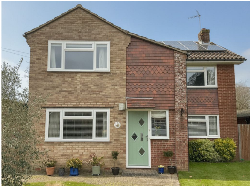
SOUTH EAST EXISTING
