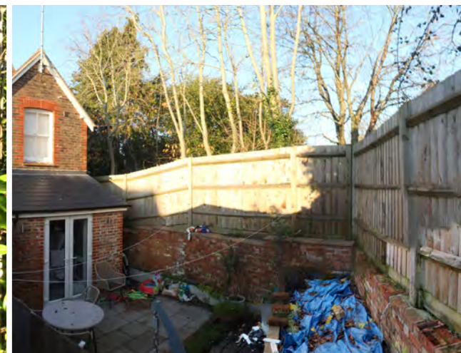
Photograph E - View of the brick retaining wall from within the existing garden to 112 Brighton Road, with treeline of the Site beyond.
