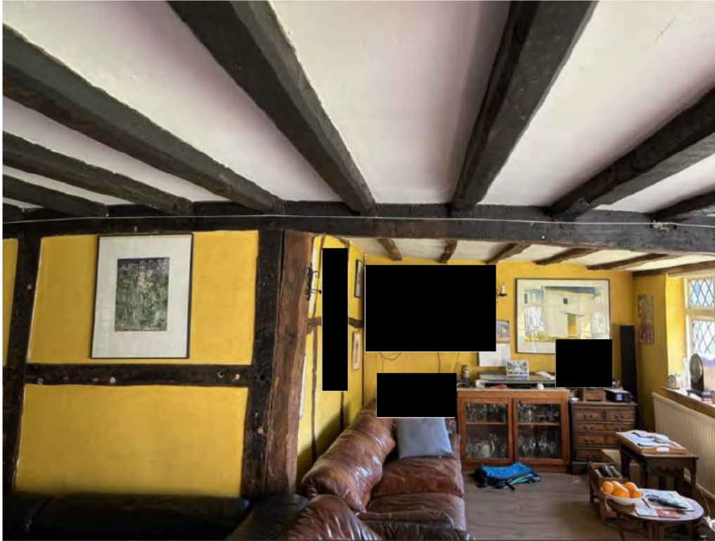
Plate 7. View of interior timber frame of Dunstans
