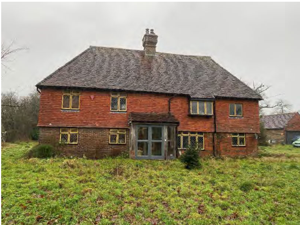
Plate 4. View of the principal elevation of Dunstons, facing north
