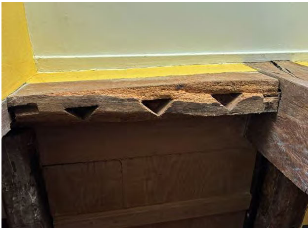
Plate 10. View of interior timber lintel inside Dunstans, showing notches from historic mullions
