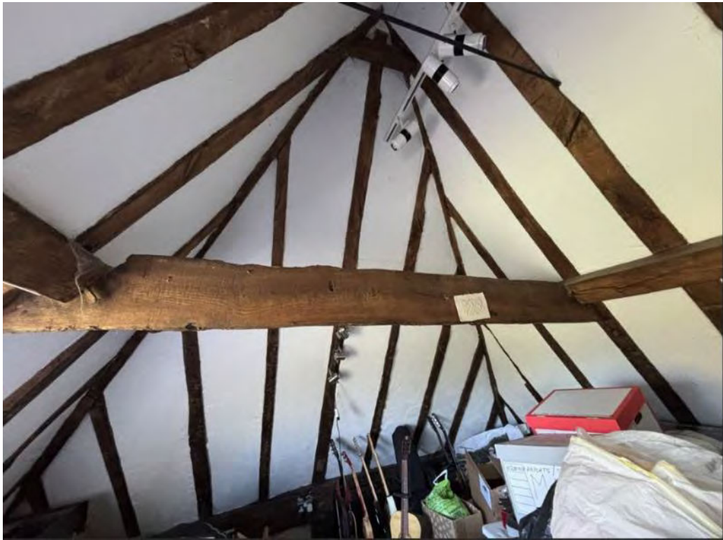
Plate 9. View of Dunstans' roof structure
