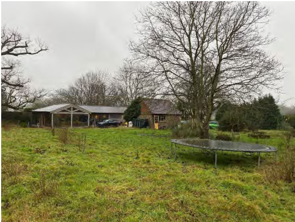
Plate 6. View of modern outbuildings at Dunstons, facing north
