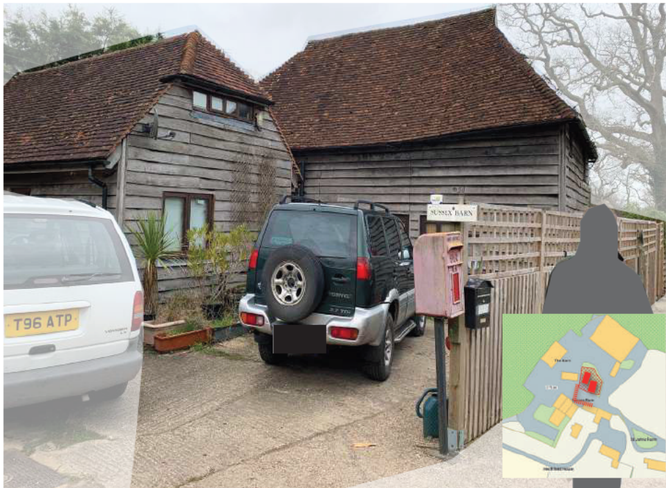
Sussex Barn - Existing converted barn to be retained excluded from application site
