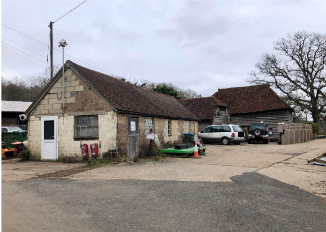
Fig 5: Sussex Barn (far right) is a former tithe barn that dates from the 17 th Century and the only historic building within the setting of the proposed site. The breezeblock building (left) is capable of replacement.
