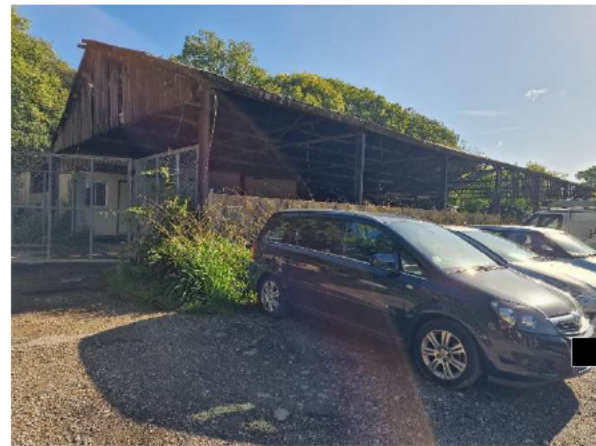
Photographs 5 and 6: Southwest corner of the building illustrating tank removal.
