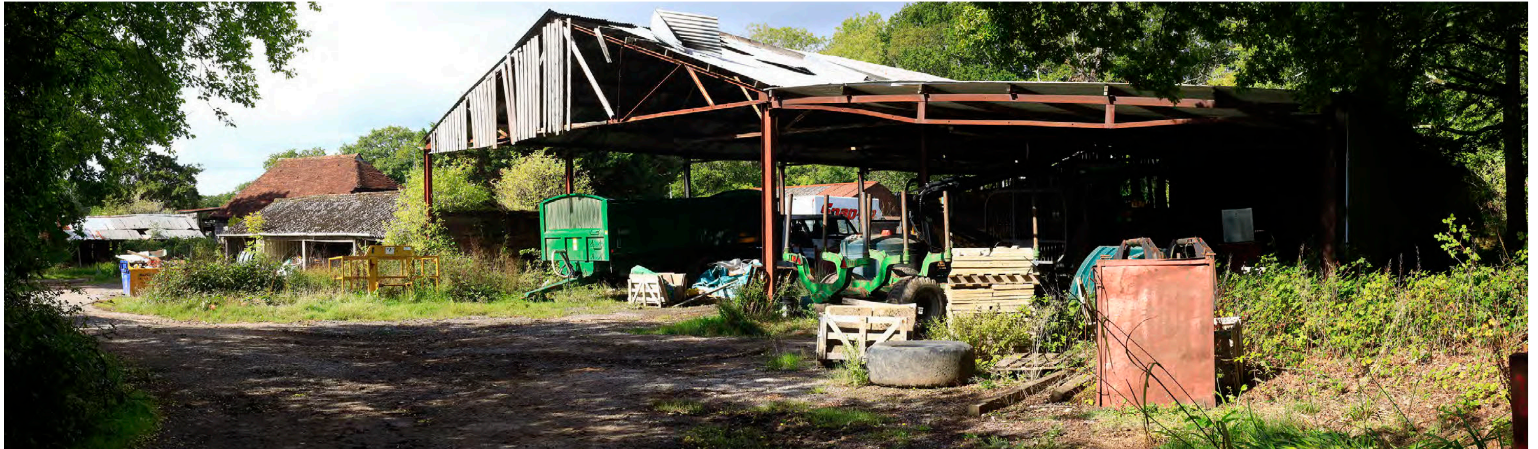
Viewpoint 07: PRoW: Footpath Looking South-West
