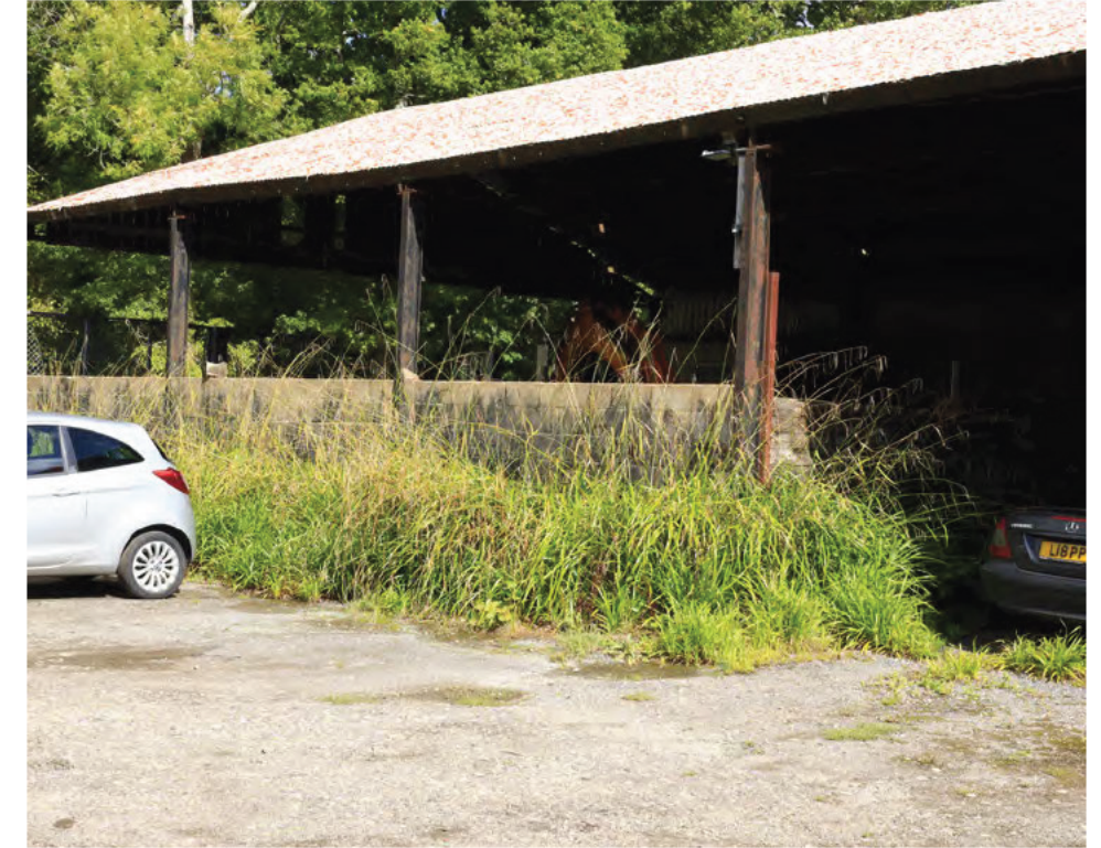
03: Open Sided Barn [Northern Edge]
