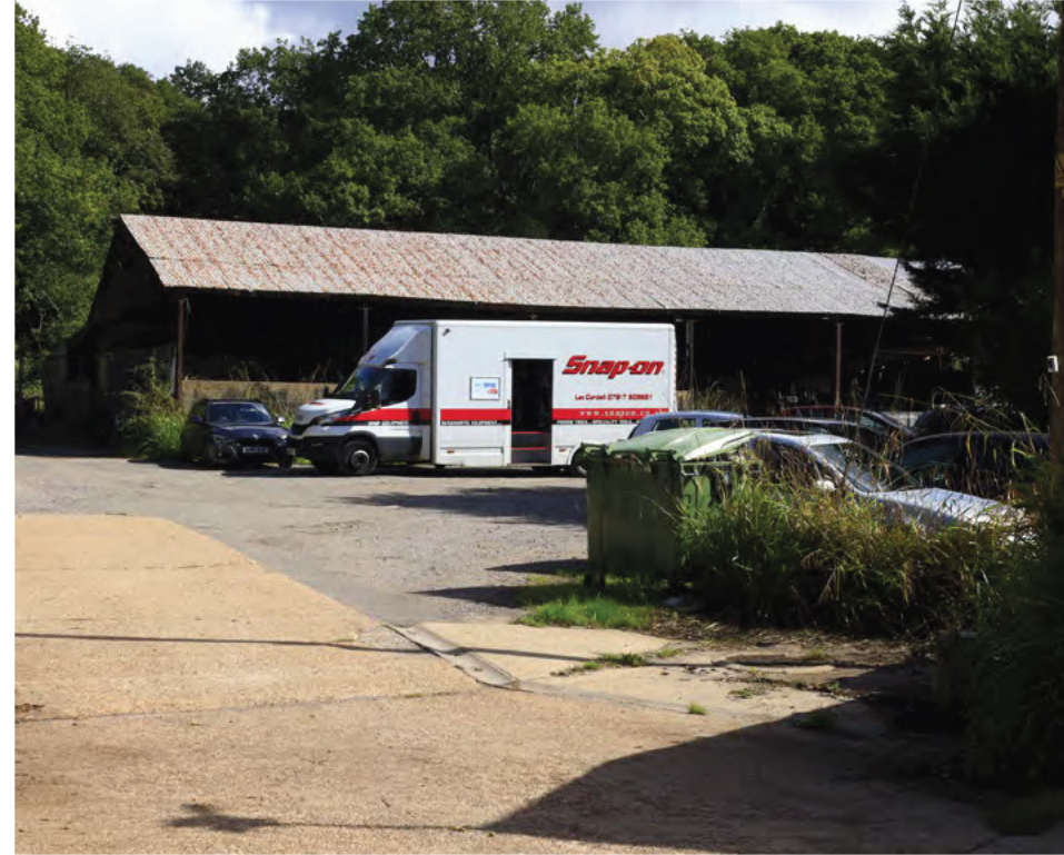
02: Open Sided Barn [Northern Edge]
