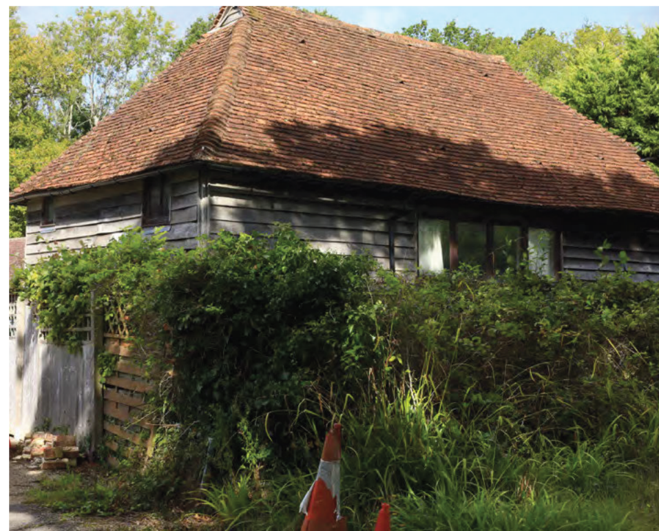
05: Sussex Barn [Previously Converted to Residential Use]
