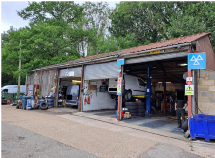
Photo 3: Displaying building B3 within the development boundary.
