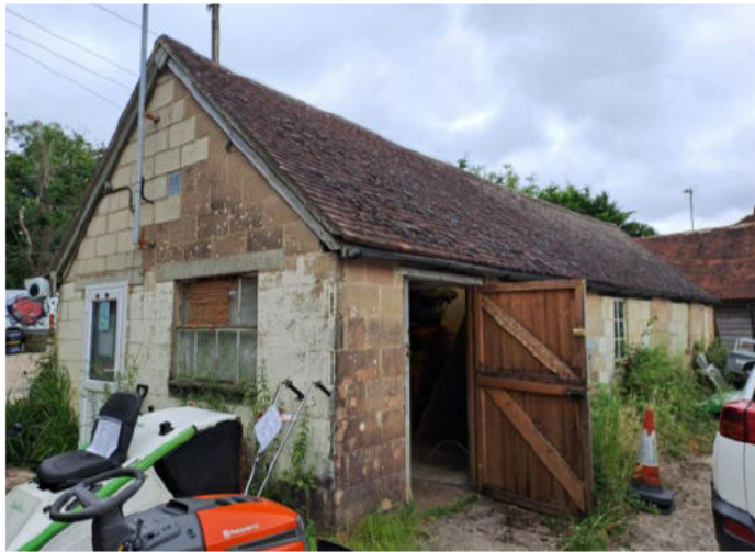
Photo 4: Displaying building B5 within the development boundary.
