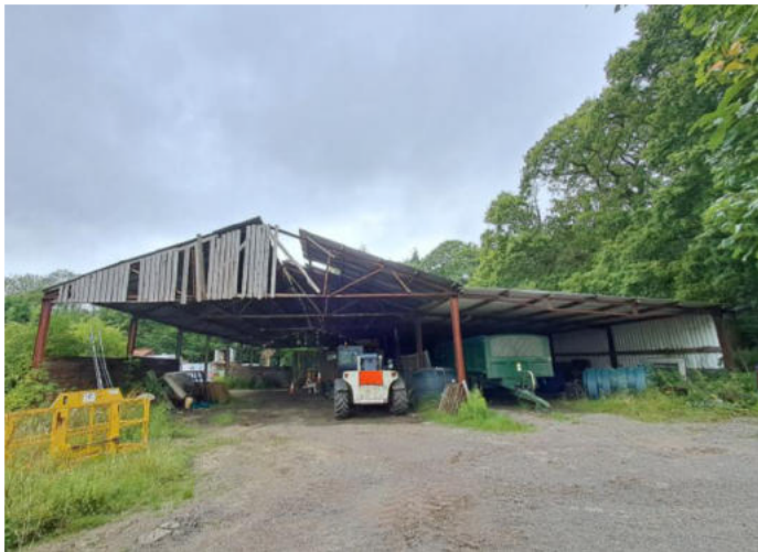
Photo 1: Displaying building B1 within the development boundary.
