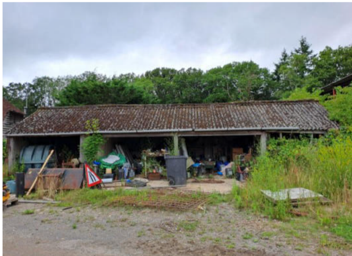
Photo 2: Displaying building B2 within the development boundary.
