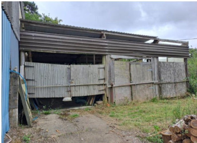
Photo 6: Displaying building B7 within the development boundary.
