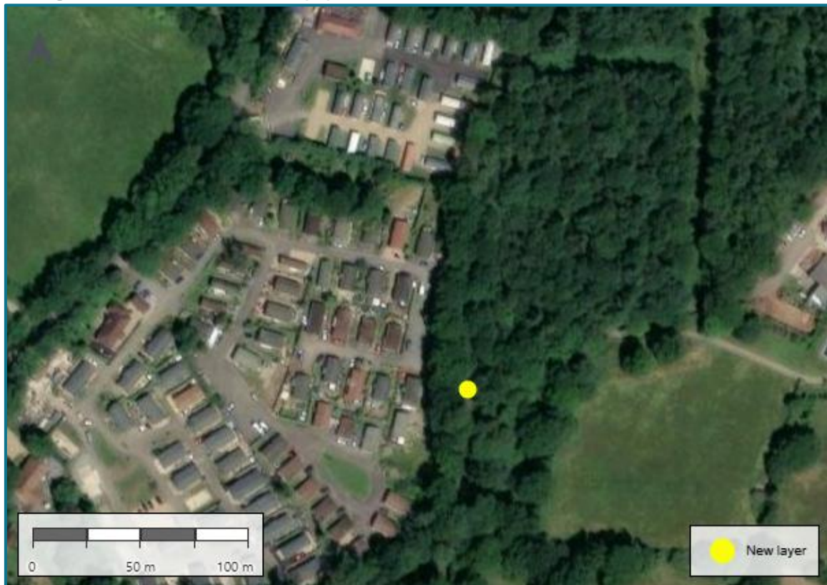
Figure 3.2 – Location of ATC Equipment
