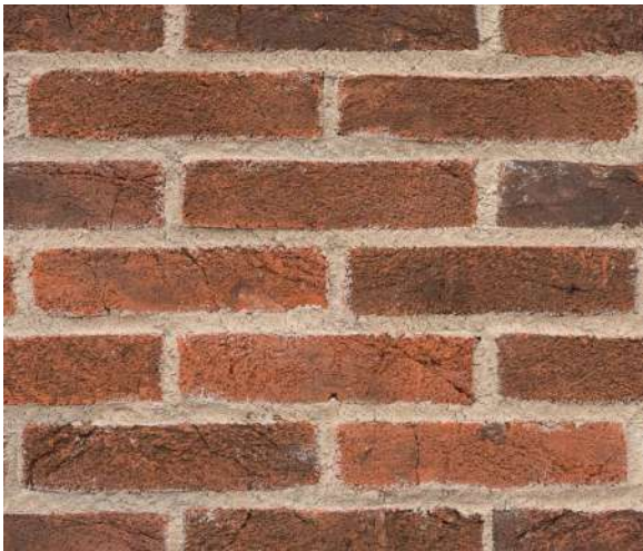
End walls and plinth walls
