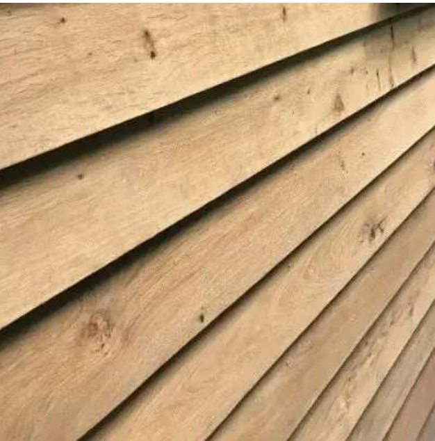
Timber external cladding
