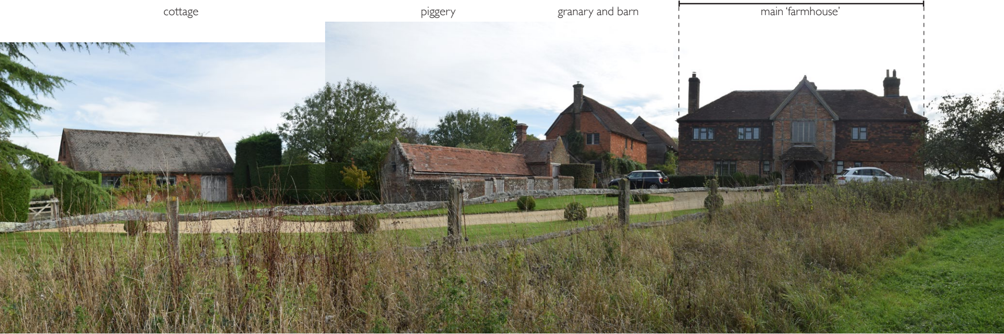
view from driveway around north of property
