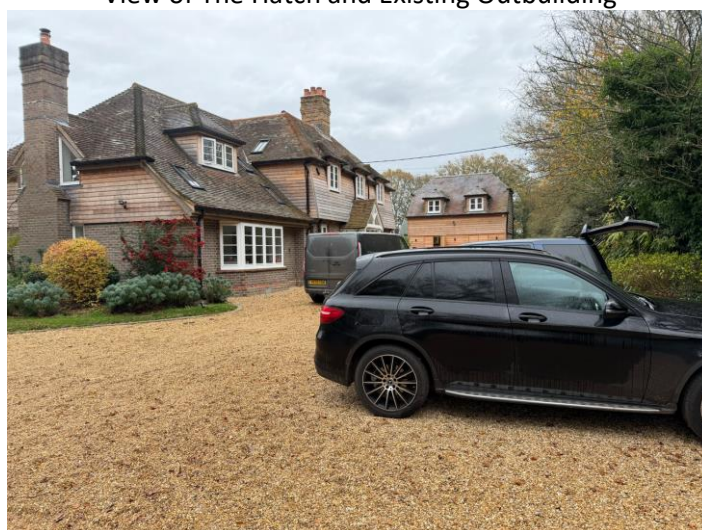
View of The Hatch and Existing Outbuilding
