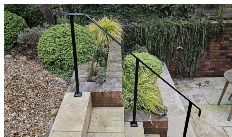
Handrails - Stepped Access
