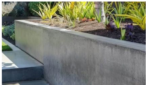
Cast In-Situ Concrete Retaining Walls
