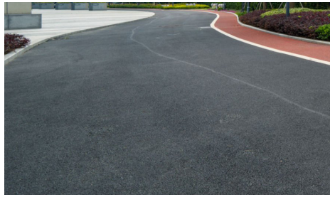
Asphalt surfacing - Pedestrian Paths
