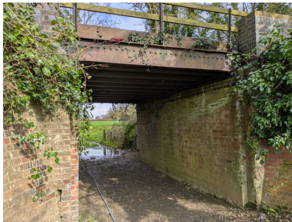
Photo 4: Southern elevation of B5.
