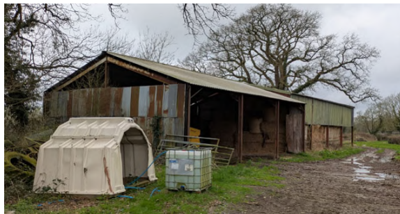
Photo 15: Northern and eastern elevations of B13 and B14.
