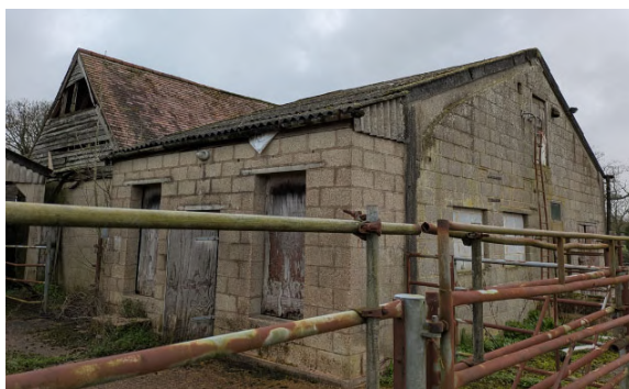
Photo 8: Eastern and northern elevations of B11 in forefront, with northern and eastern elevations of B12 in rear of photo.
