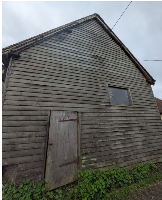
Photo 11: Western elevation of B12.
