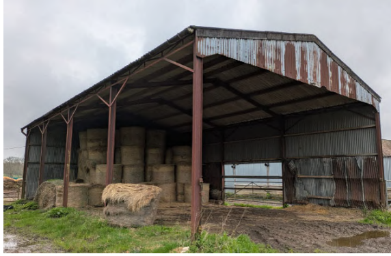
Photo 5: Northern and eastern elevations of B8.
