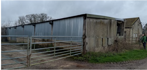
Photo 6: Northern and eastern elevations of B9, with B11 in right side of photo.
