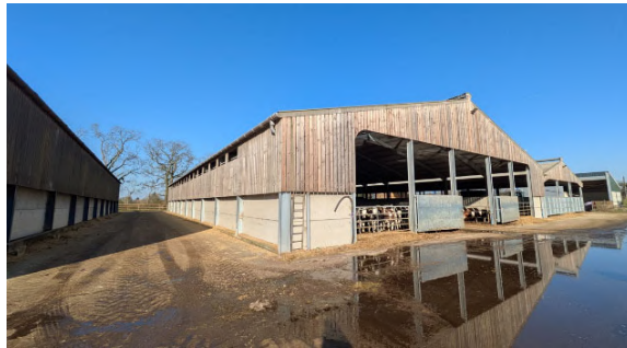
Photo 2: Southern and eastern elevations of B3 in the centre of the image, with northern elevation of B4 in left-side of photo and southern and eastern elevations of B2 and B16 in right side of photo.
