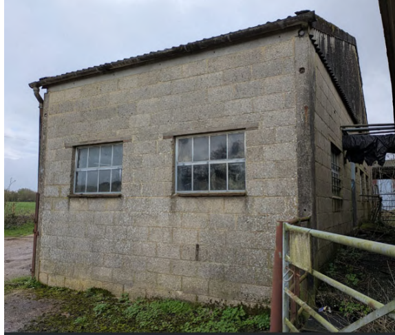
Photo 9: Southern and western elevations of B11.
