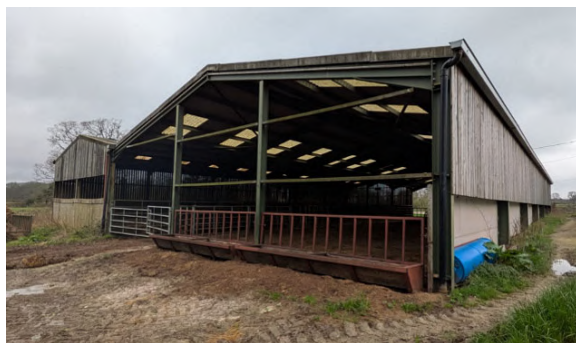
Photo 16: Southern elevation of B15.
