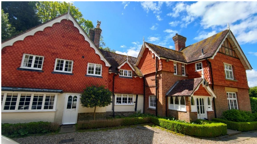
Fig.10 photo of the existing front elevation
