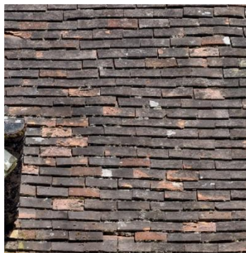
Fig.13 The existing roof finish
