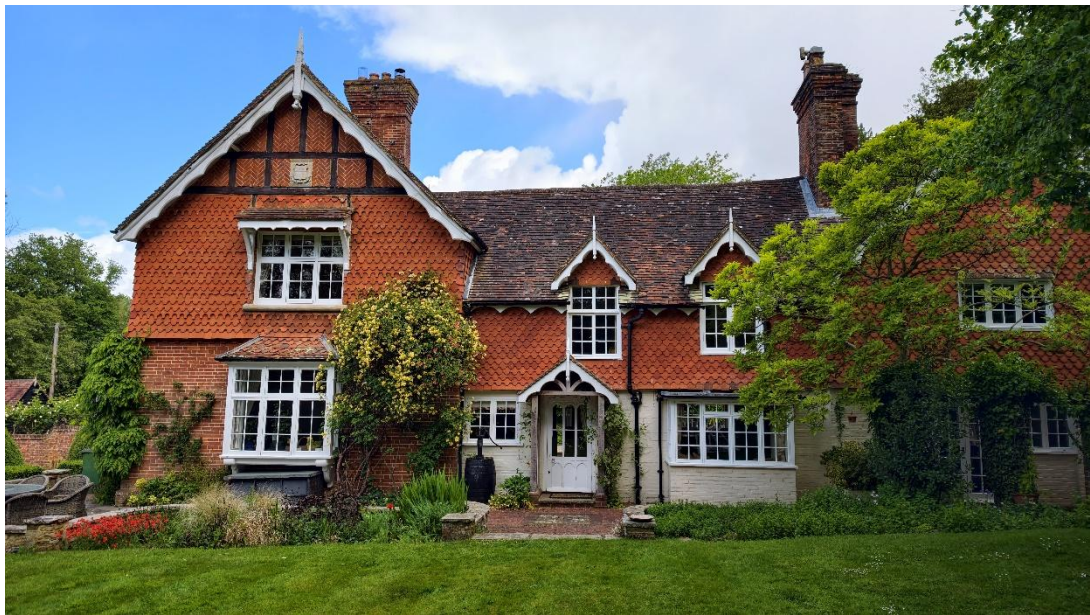
Fig.11 photo of the existing rear elevation
