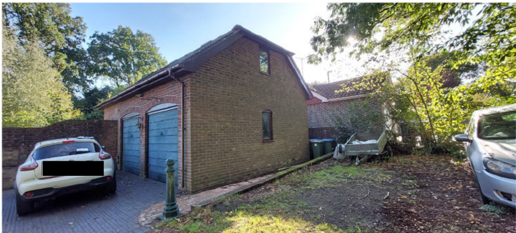
Photograph No: 7 – View of B02 showing well-constructed building with a couple of small gaps but no obvious PRFs
