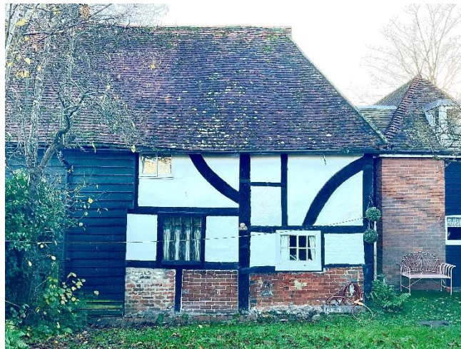
Figure 2. Rapley Cottage north elevation (rear) showing original timber framing.
