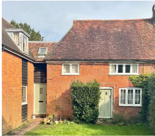
Figure 3. Rapley Cottage south elevation (front) showing later C18 brick frontage
