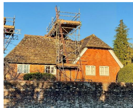
Patchings Grade II
