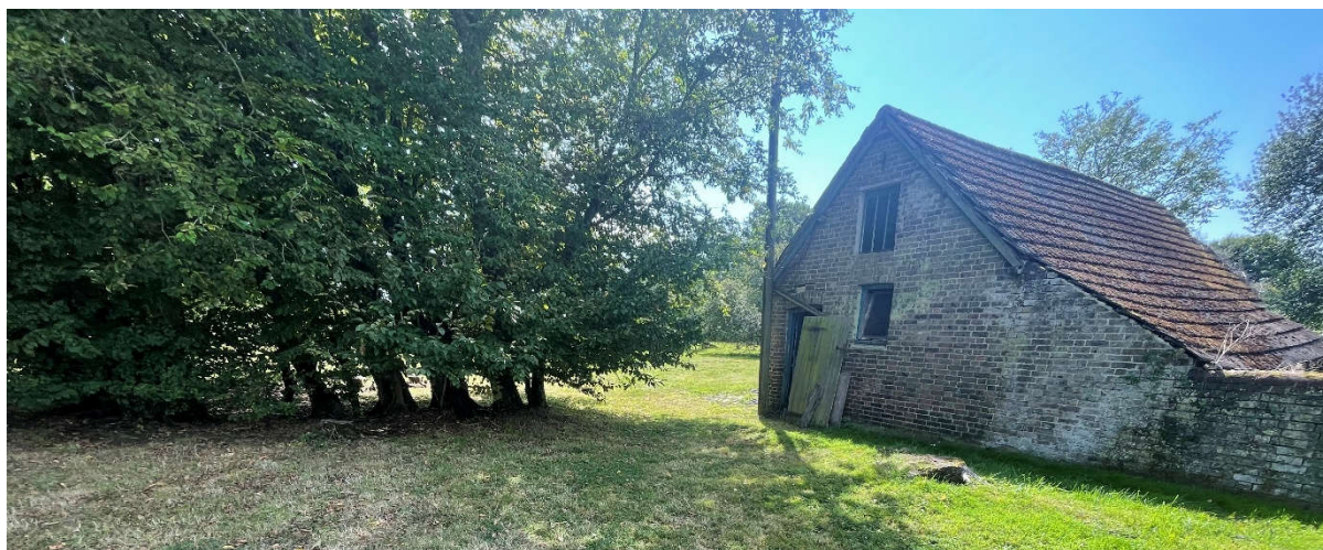
Trees close to north-east corner of building
