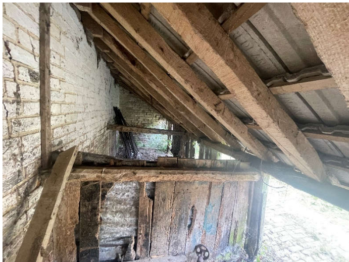
Lean-to roof structure
