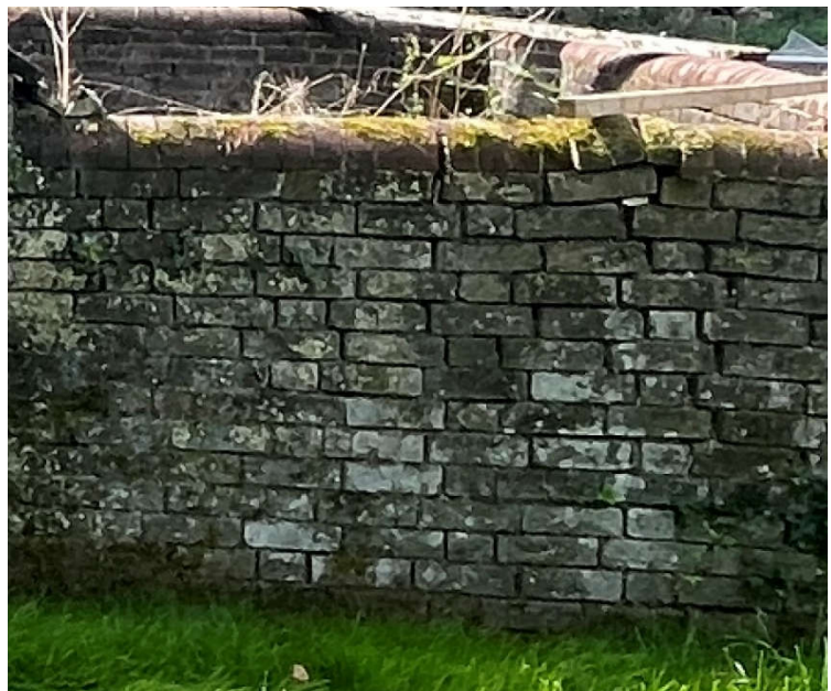
Typical condition of boundary wall to yard
