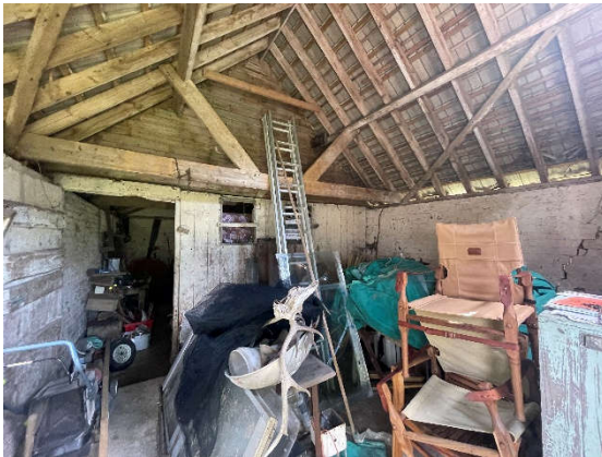
Roof structure at South end of building
