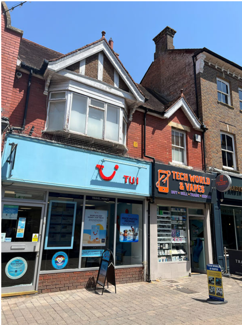
56A & 56B West Street - front view
