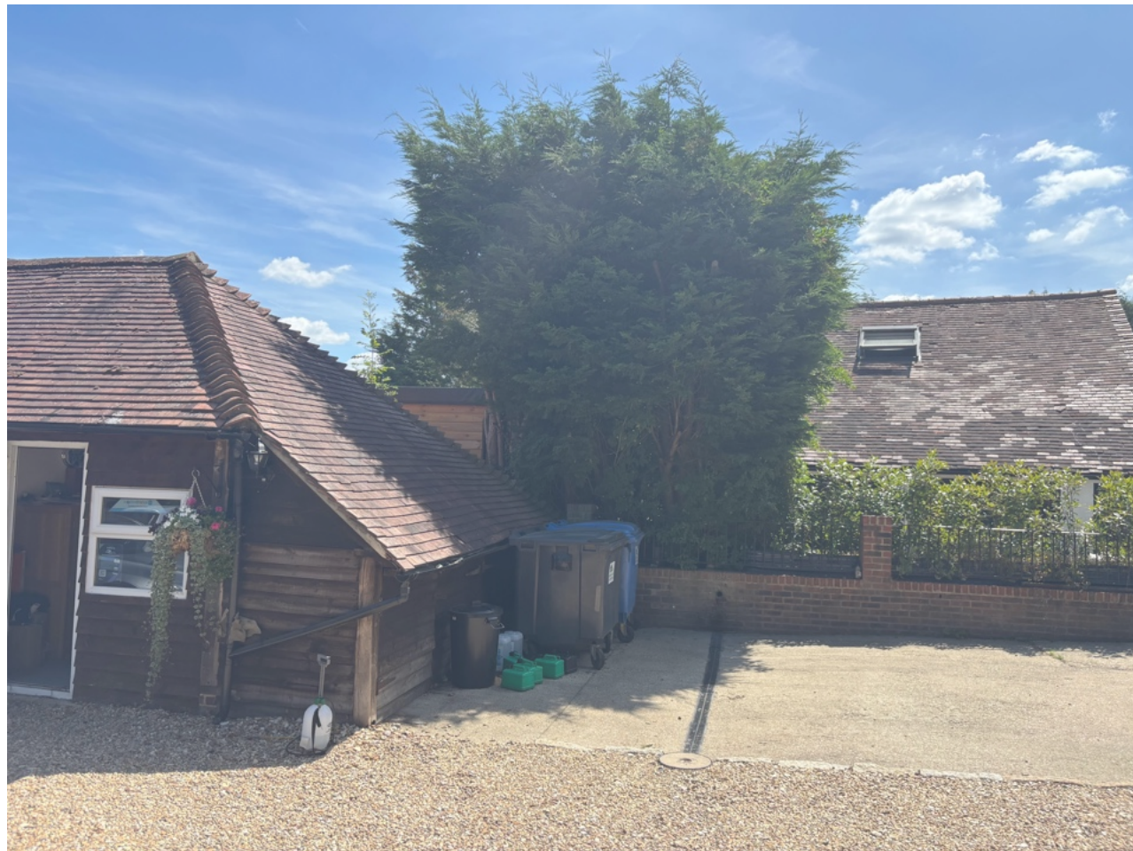
3. VIEW TOWARDS ADJOINING SITE
