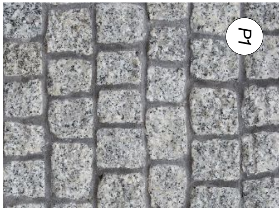
P1 PERMEABLE PAVERS
