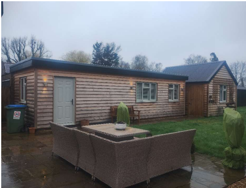
Existing (As-Built) Garden Annex and Workshop
