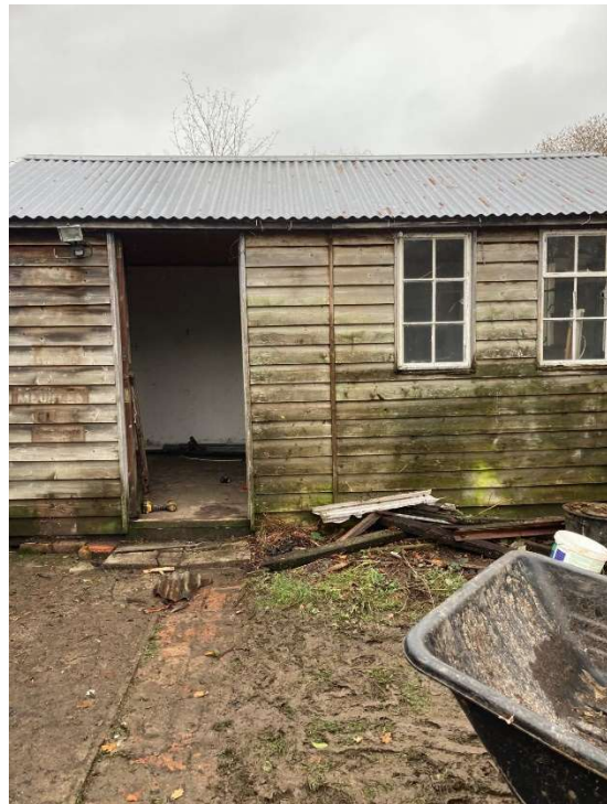
Pre-Existing Outbuilding (workshop)
