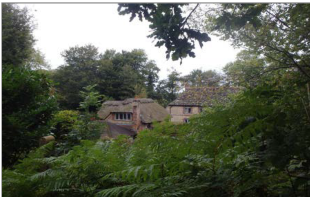
Plate 7.6: View of East Wantley farmhouse (11) through a gap in the trees from the public footpath to the north-west of the Site (looking north-east)
