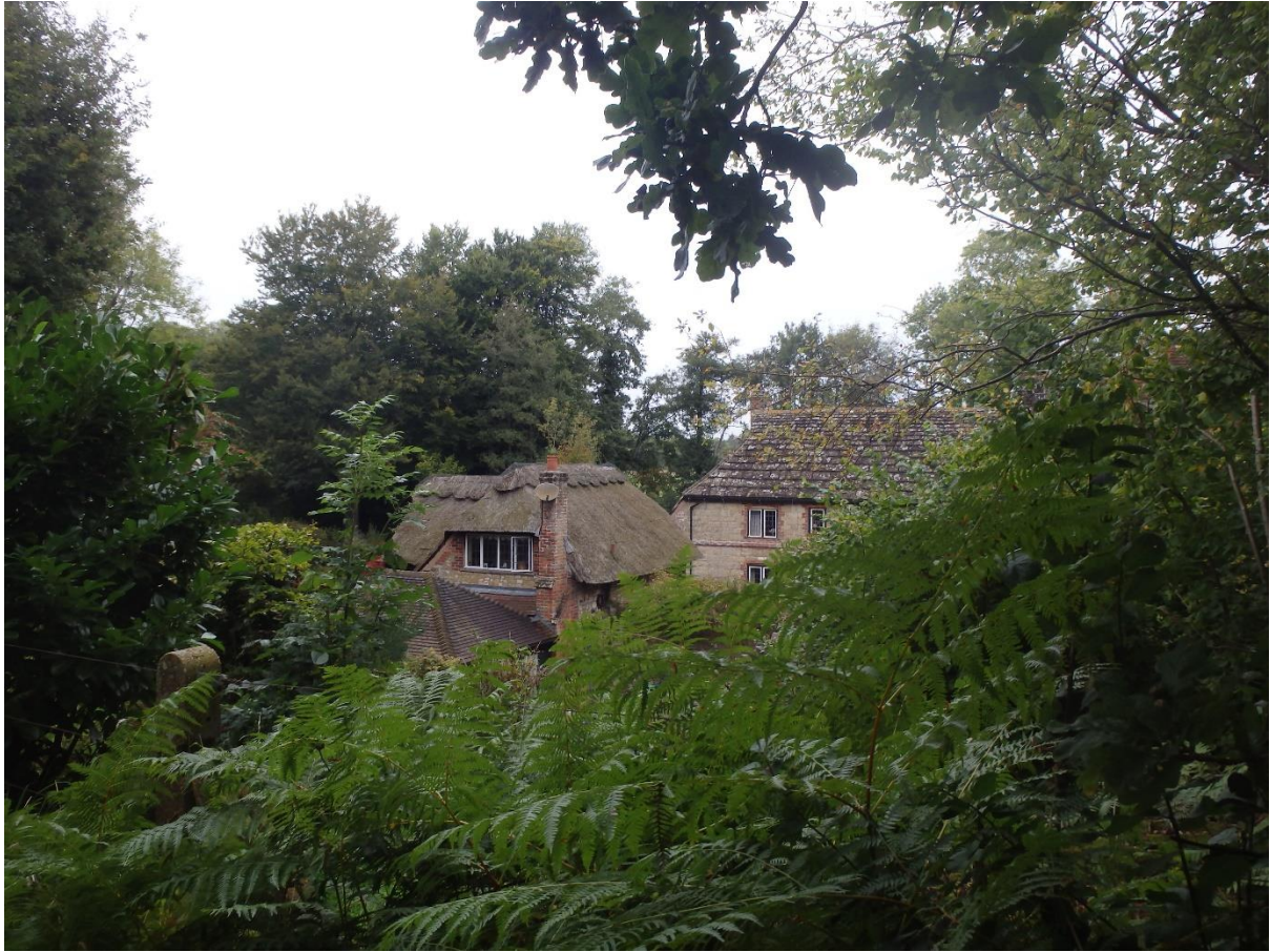
Plate 9: East Wantley (right) facing north-west from the north public footpath (archive photograph dated 2017).
