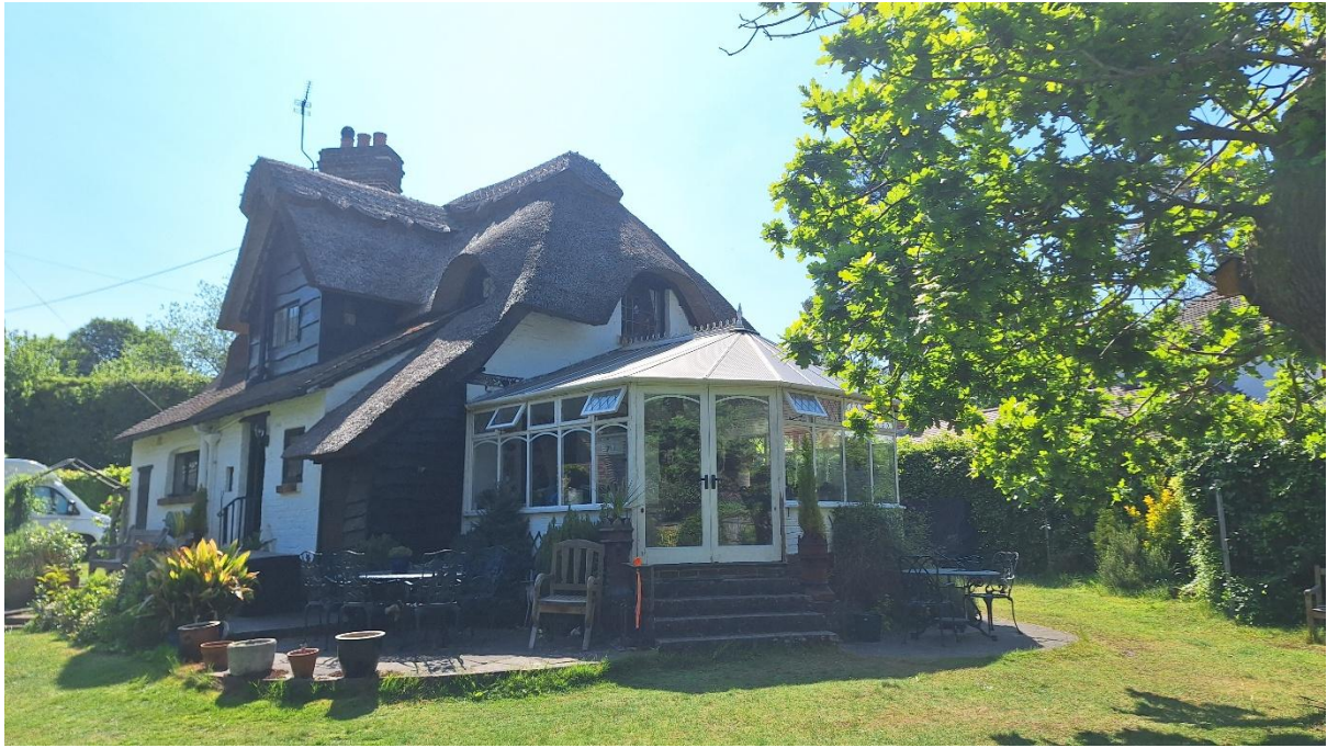
Rear view of main cottage, showing modern conservatory addition.
