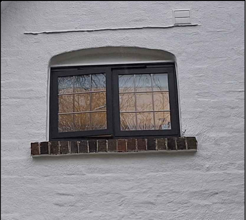
Slimline DG aluminium framed glazing in timber subframes.
