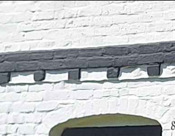
Painted masonry, dentil courses & arched heads to openings.
