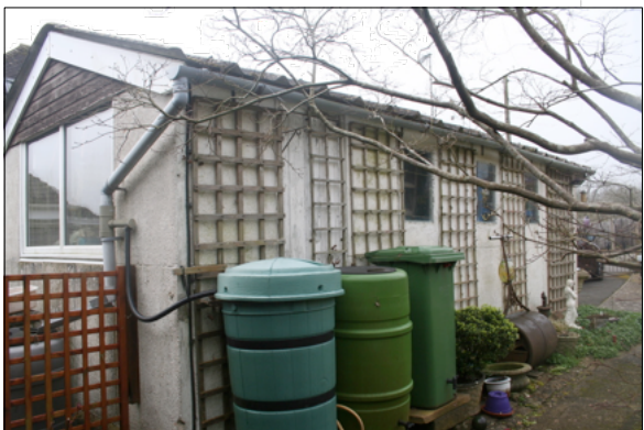
South side elevation of garage
