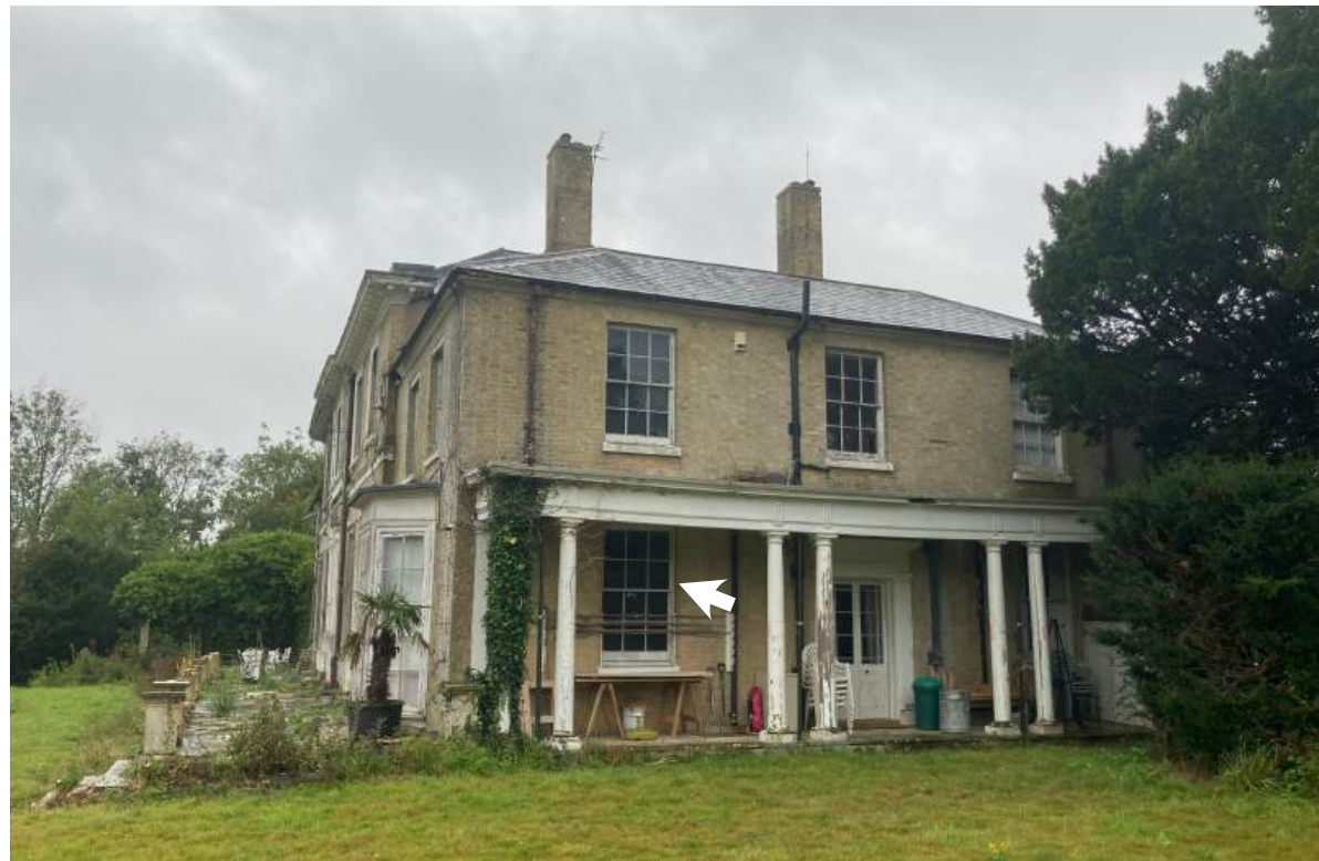
Blocked window to be reinstated.
