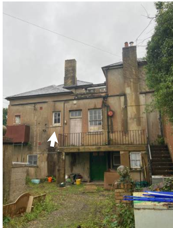
Window to be widened.
