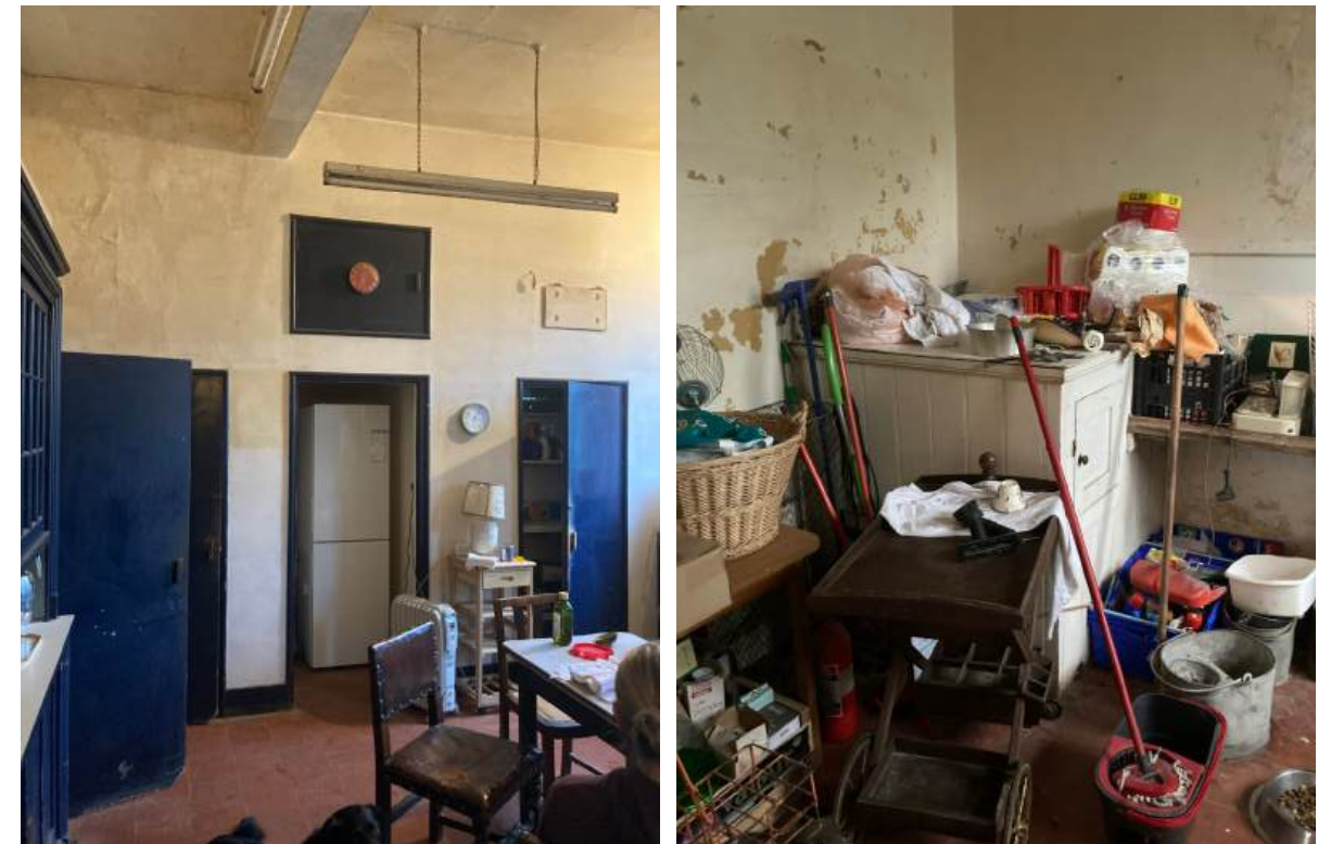
Existing pantry and coal stores to be removed/altered and worktop and basin to be removed.
