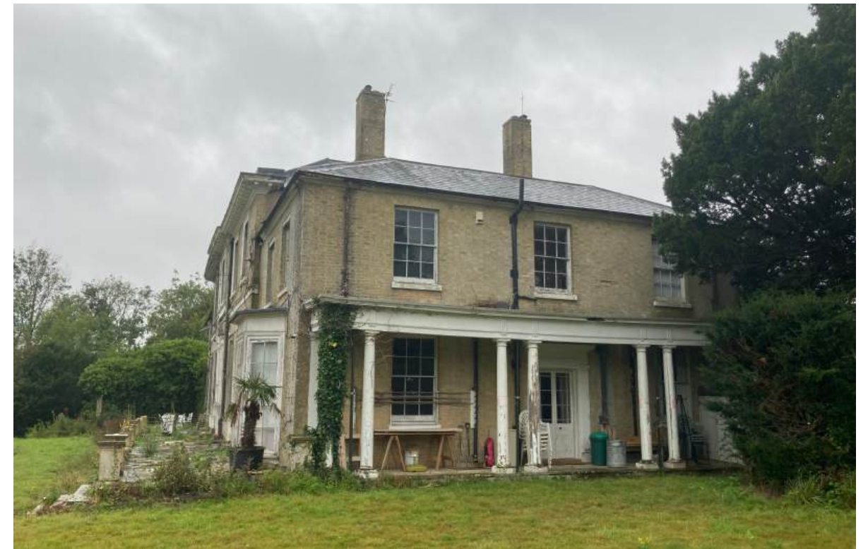
Existing veranda to be rebuilt.
