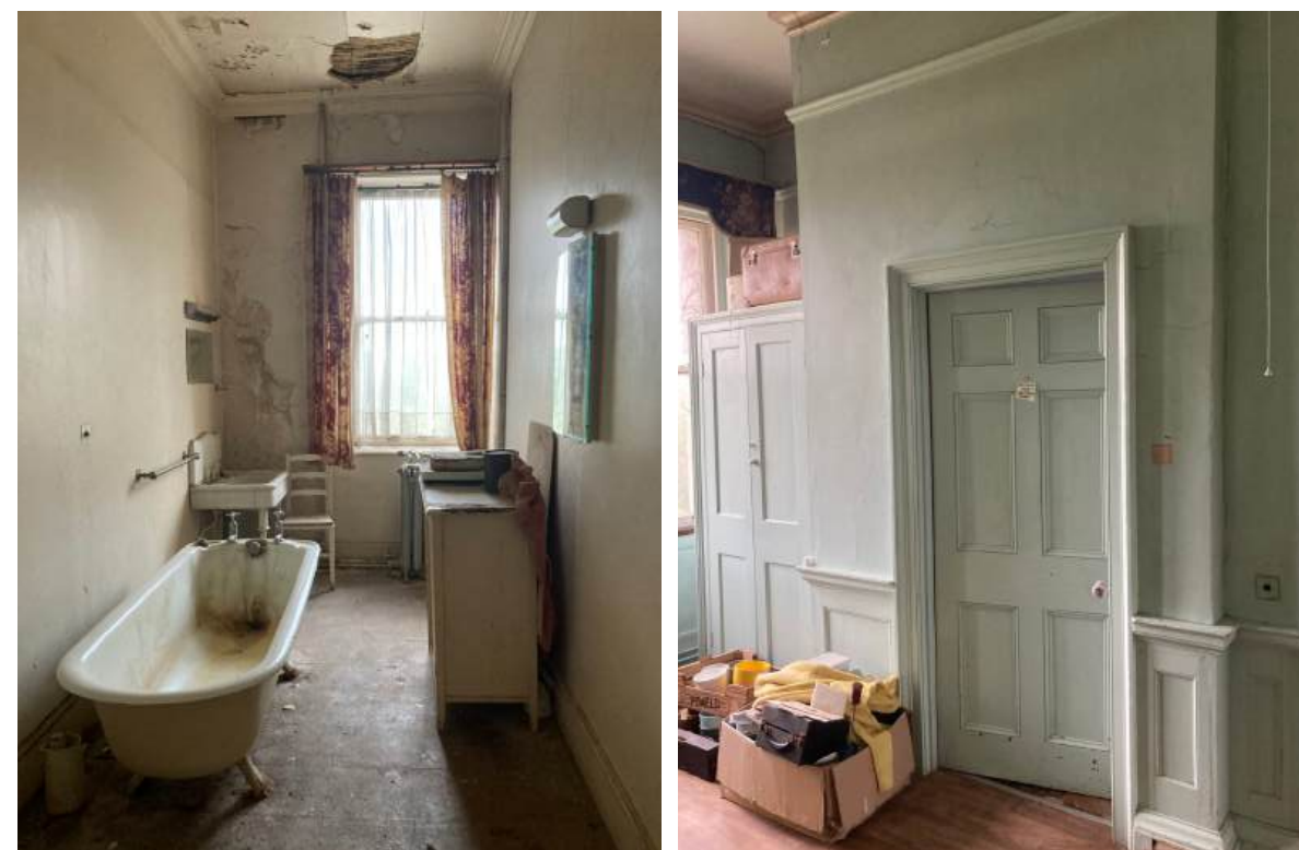
Bathroom to be refitted with historic bathtub and sink retained. Modern opening in chimney breast to be blocked.
