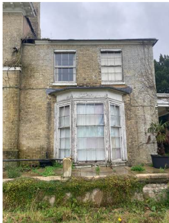
Bay window to be altered.
