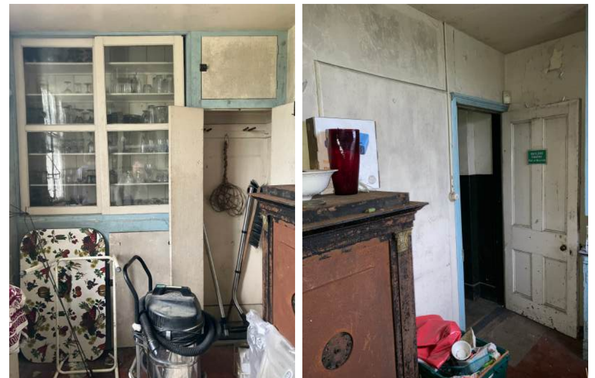
Mid-20 th century cabinetry and partitions to be removed.
