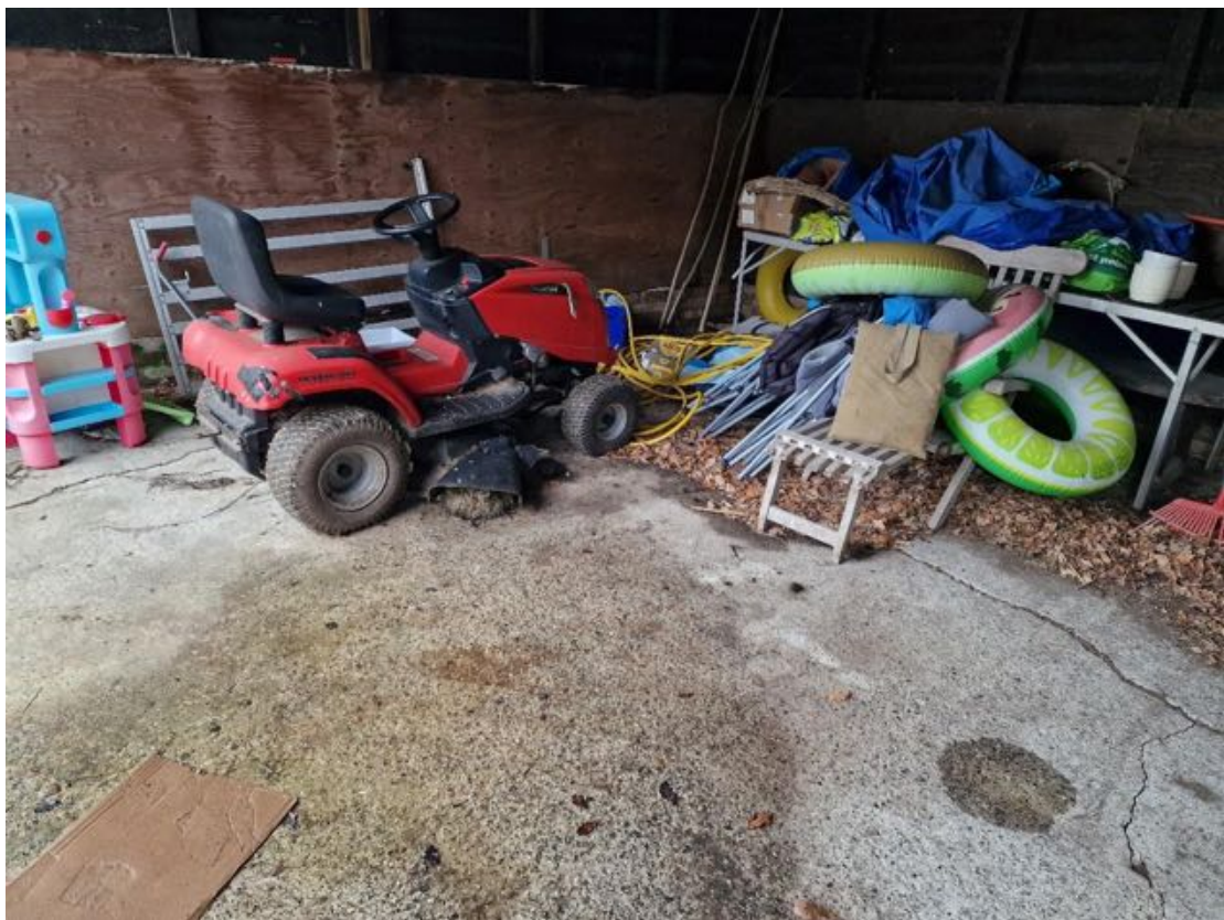
Garage concrete surfacing
