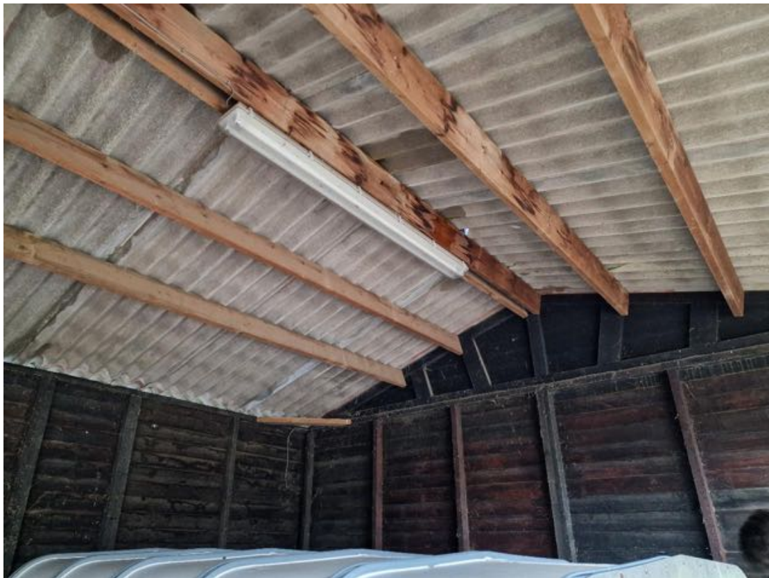
Garage roof roofing
