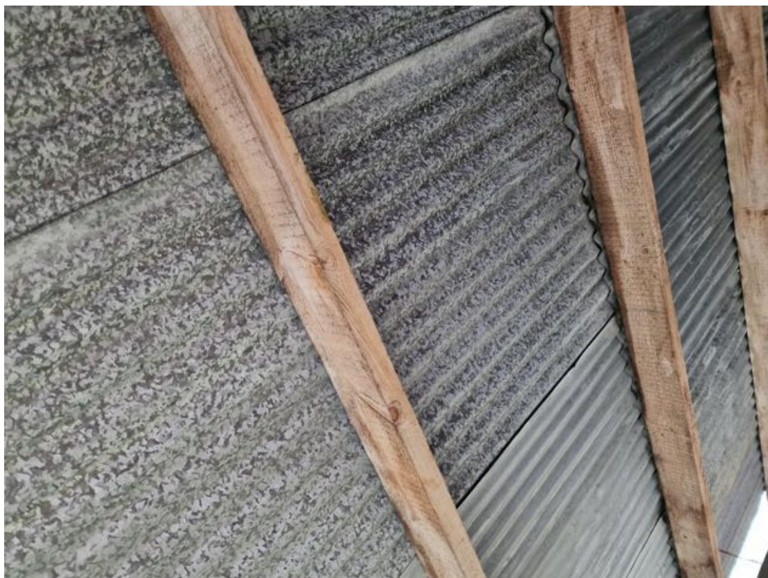
Machinery store roofing
