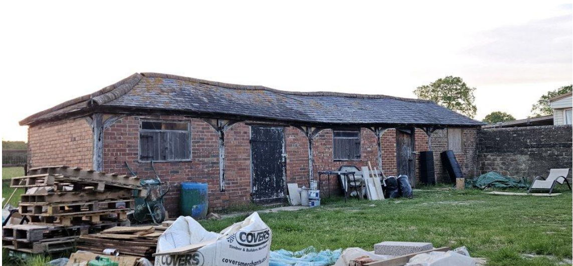
Figure 4: Outbuilding B1 east elevation
