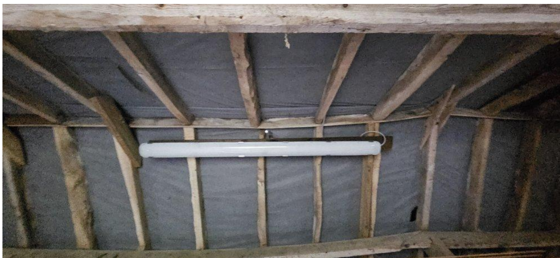
Figure 7: Outbuilding B1 internal central roof area
