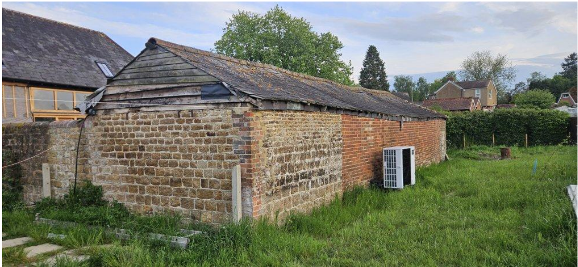
Figure 2: Outbuilding B1 north elevation
