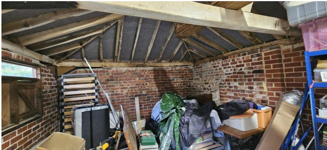
Figure 6: Outbuilding B1 internal space facing south
