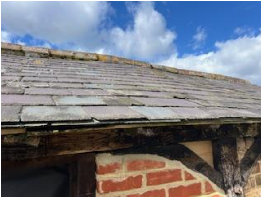
Photo 3 – Detail of B1 roof.
