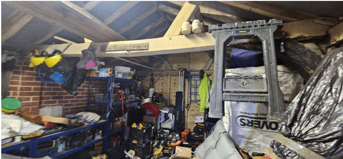
Figure 5: Outbuilding B1 internal space facing north
