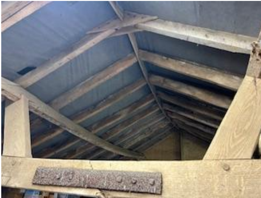
Photo 5 – Inside of B1.
