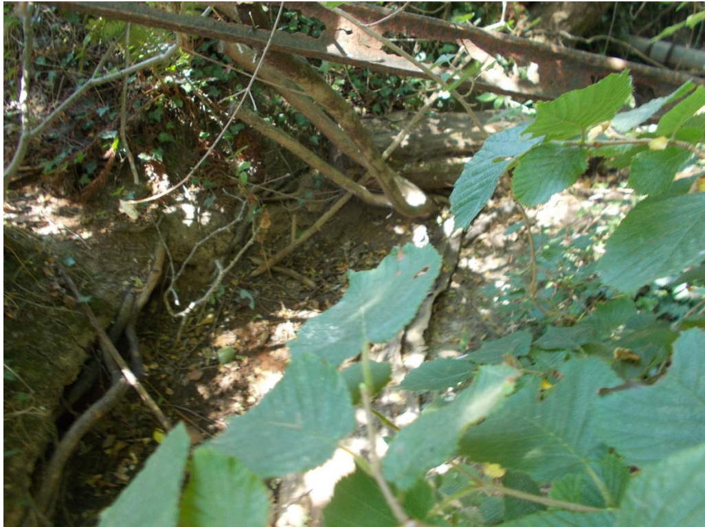
Photo 3: Junction where roadside drainage ditch joins boundary ditch.
