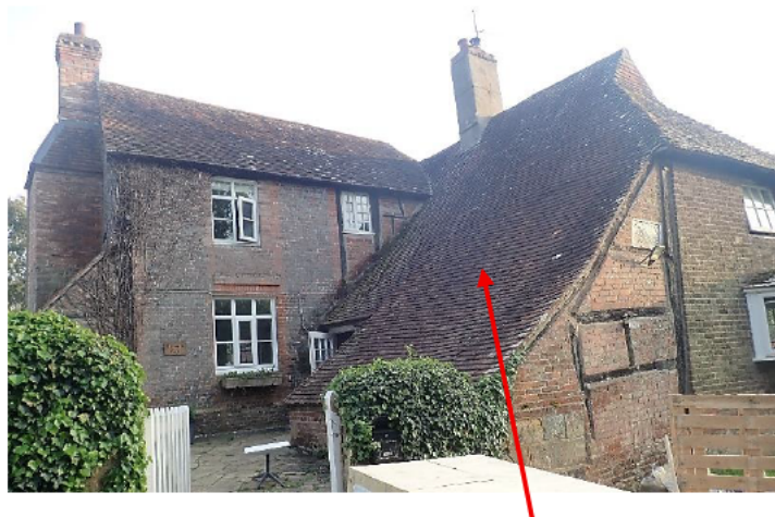
Fig. 5 – The house, viewed from the NE – catslide roof to be renovated
