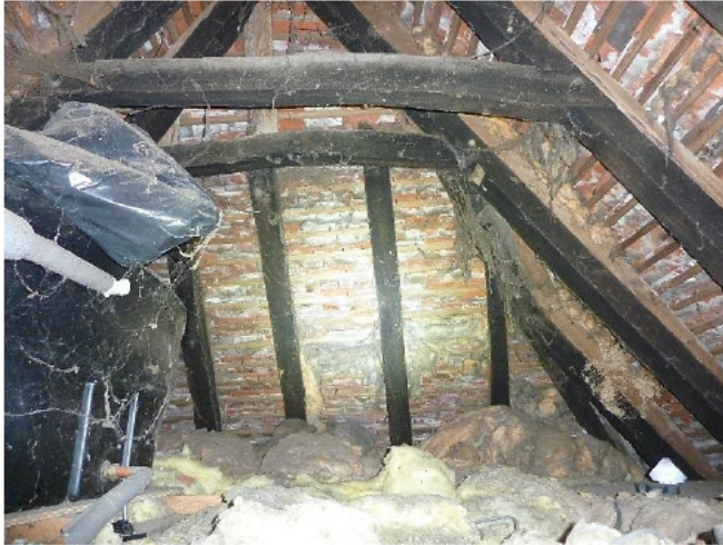
Fig. 9 – Unlined roof in older section of building (N/S)
