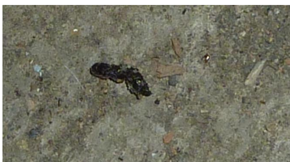
Fig. 7 - Bat dropping on floor of E/W roof void
