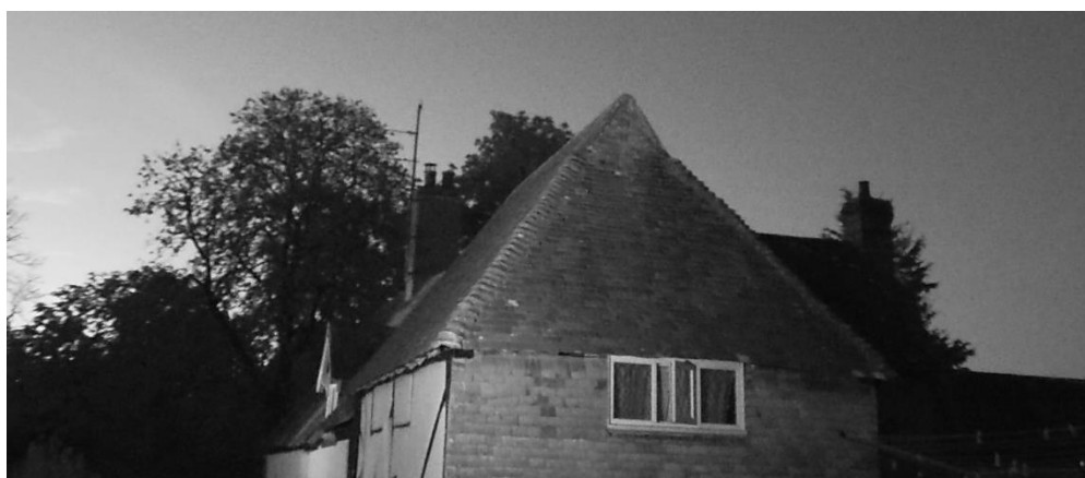
Fig. 19 – IR camera view from S, Survey 2
