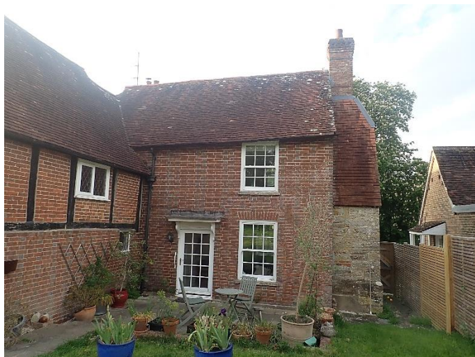
Fig. 6 – The house, viewed from the SE
