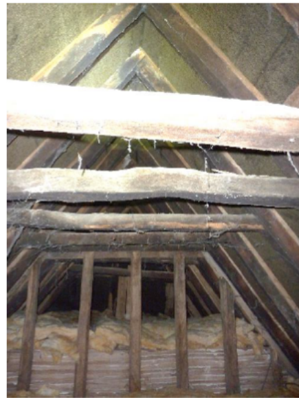
Fig. 10 – Lined section of roof, to south
