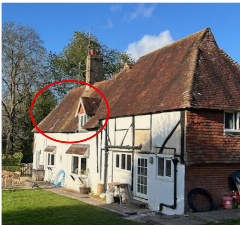
Fig. 1 – New dormer window to be fitted to left of existing dormer, replacing old skylight window This section of roof (NW) to be re-tiled (Property owner's photograph)
