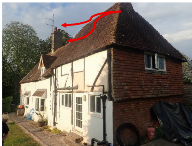
Fig. 18 – Svy 1 - Emergence point of two pipistrelles, S end roof
