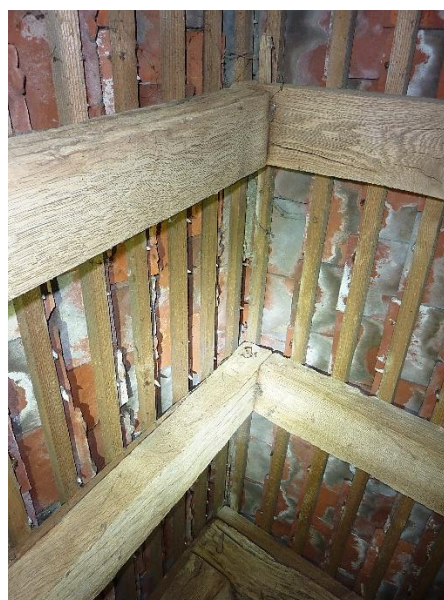
Fig. 8 – Unlined section of roof (E/W section)
