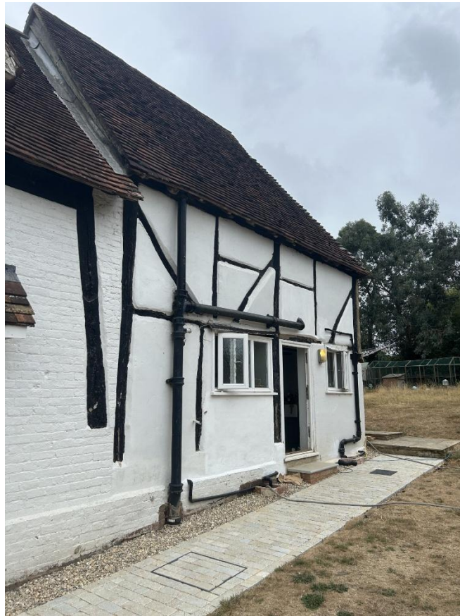
Fig 20: photo of the existing west elevation, southern end of range
