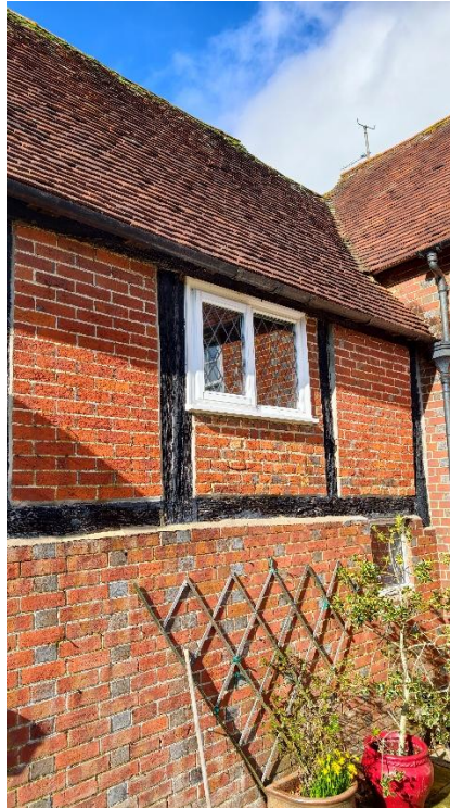
Fig 16: photo of the existing east elevation, southern end of long range
