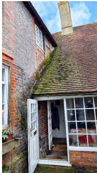
Fig 14: photo of the existing east elevation, entrance porch
