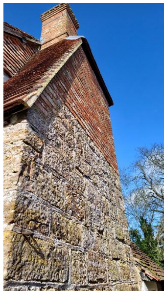
Fig 15: photo of the existing east elevation, eastern chimney
