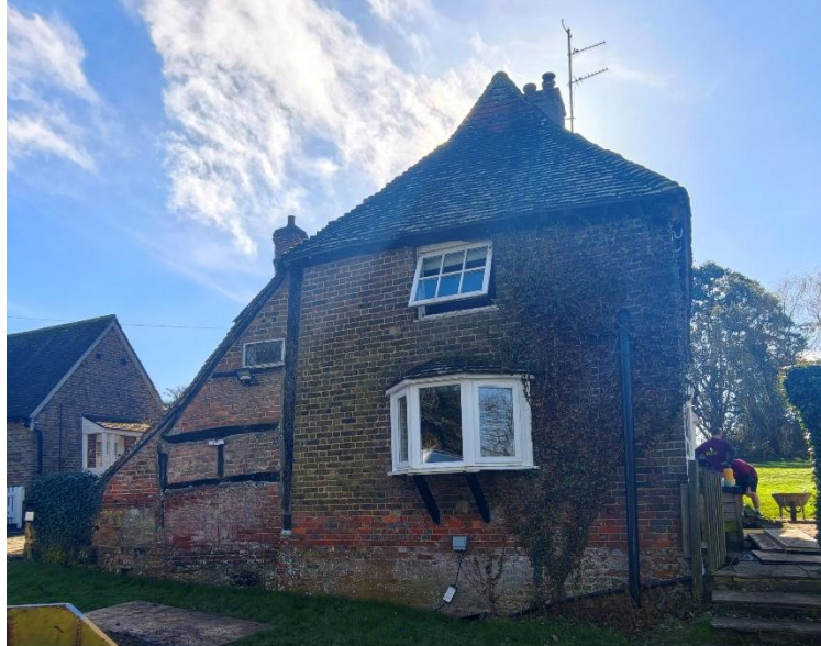
Fig 12: photo of the existing north elevation, northern end of long range
