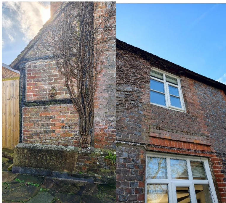
Fig 13: photo of the existing north elevation, eastern range
