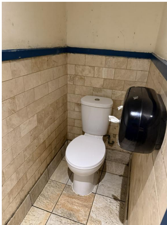
Photography: Existing Male WC's to be refurbished
