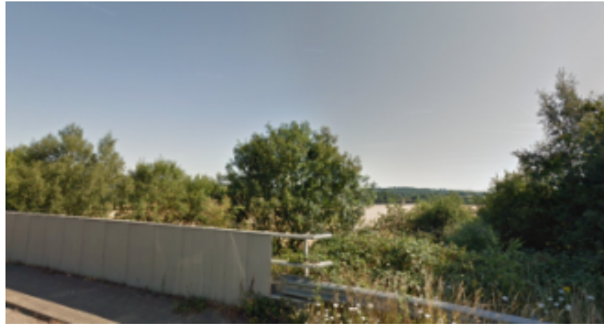
Street View - A264 Railway Bridge looking North
