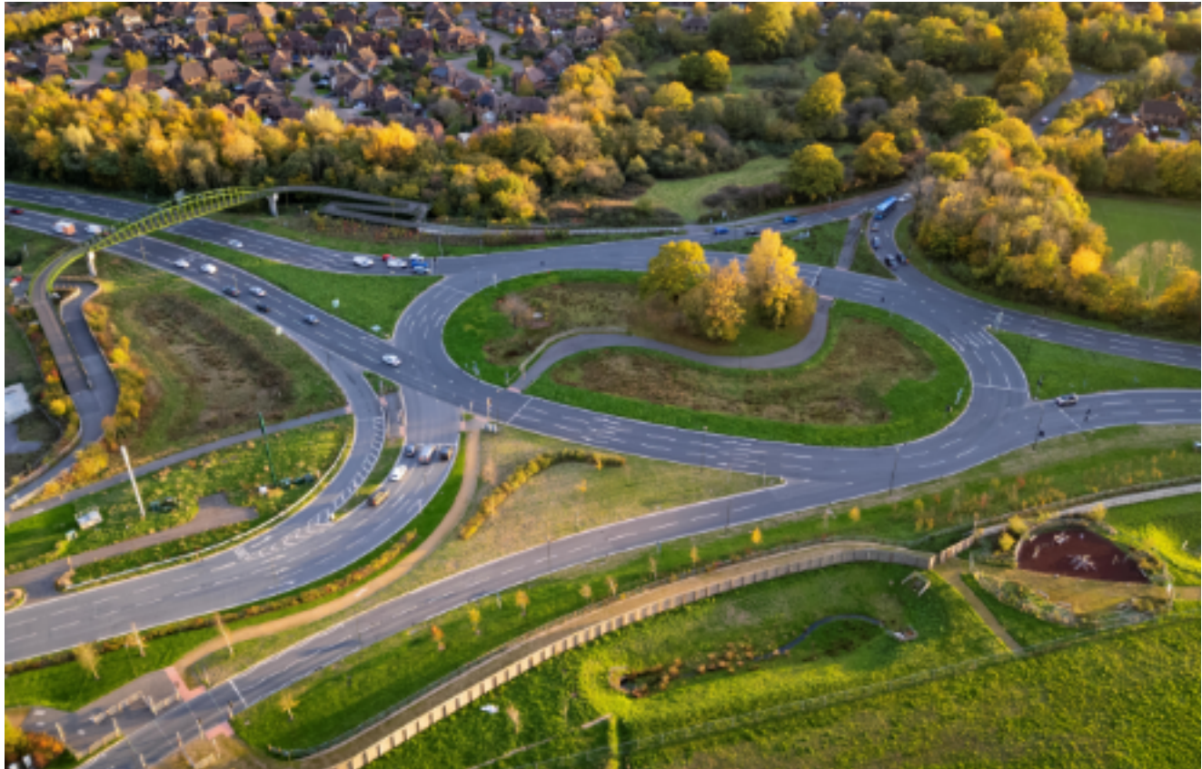
Aerial View - Completed Rusper Roundabout looking East towards the employment land
