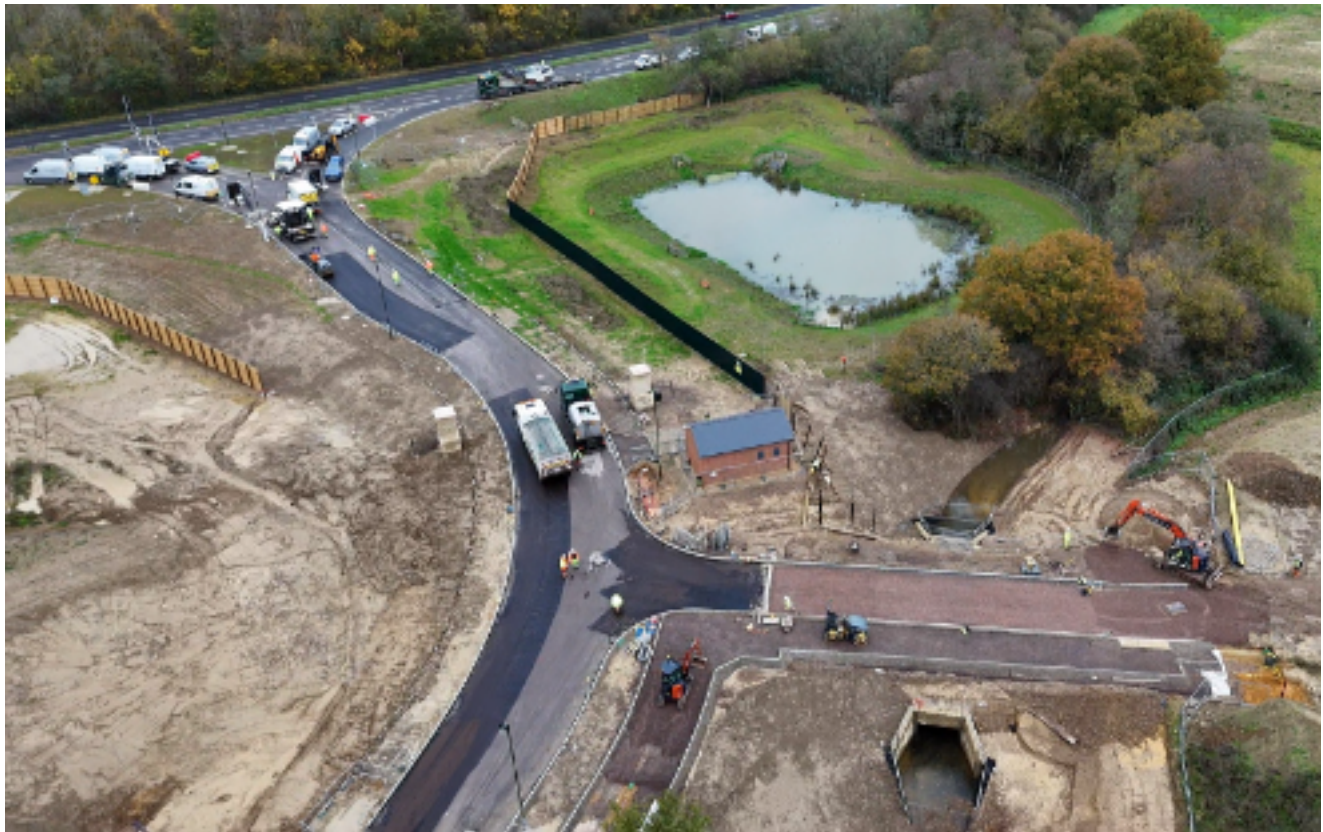
Aerial View - New LiLO under construction for access to Employment Land and the new sports hub
