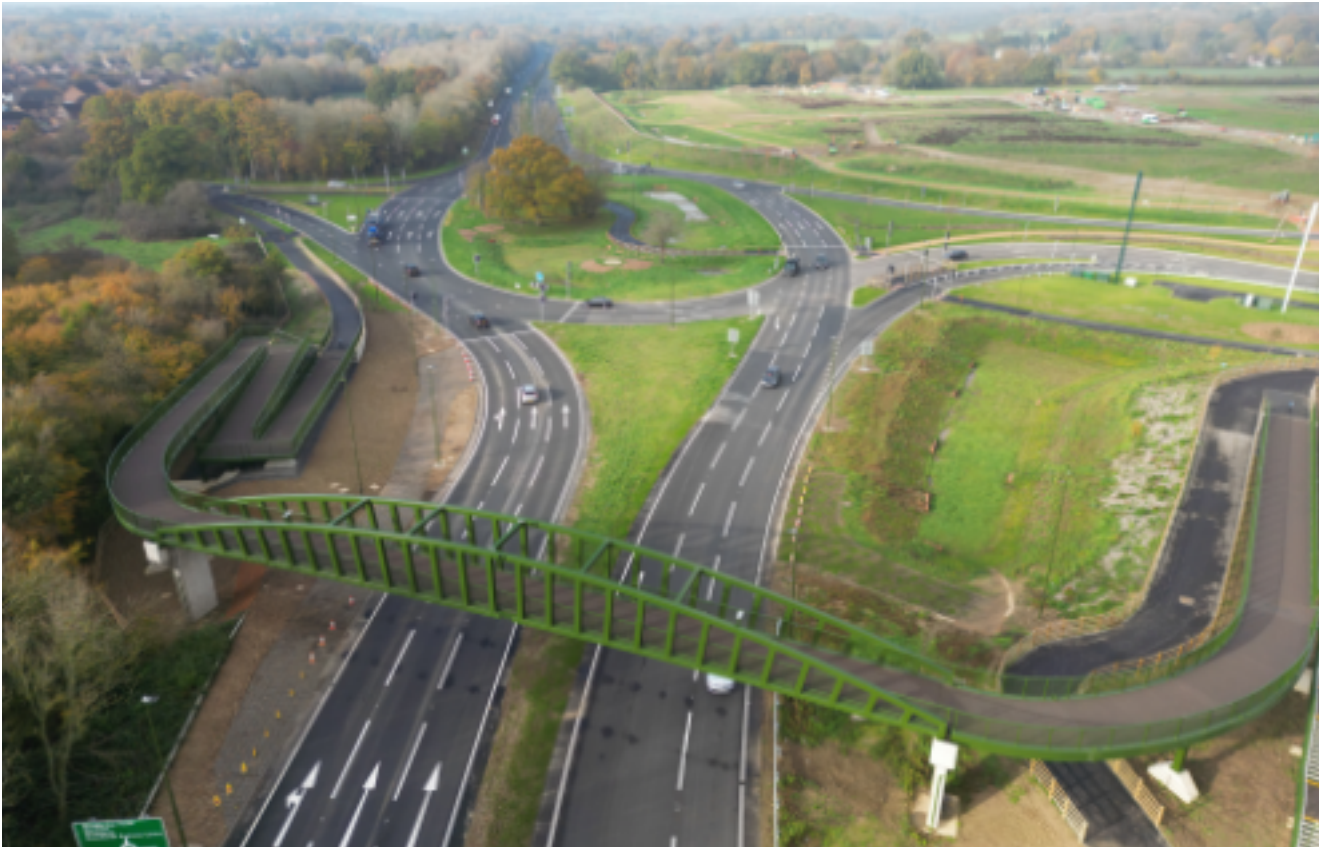
Aerial View - Completed Rusper Road roundabout looking West
