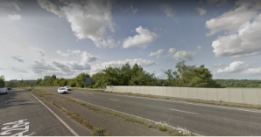
Street View - Road from SE along A264 over railway bridge looking NW
