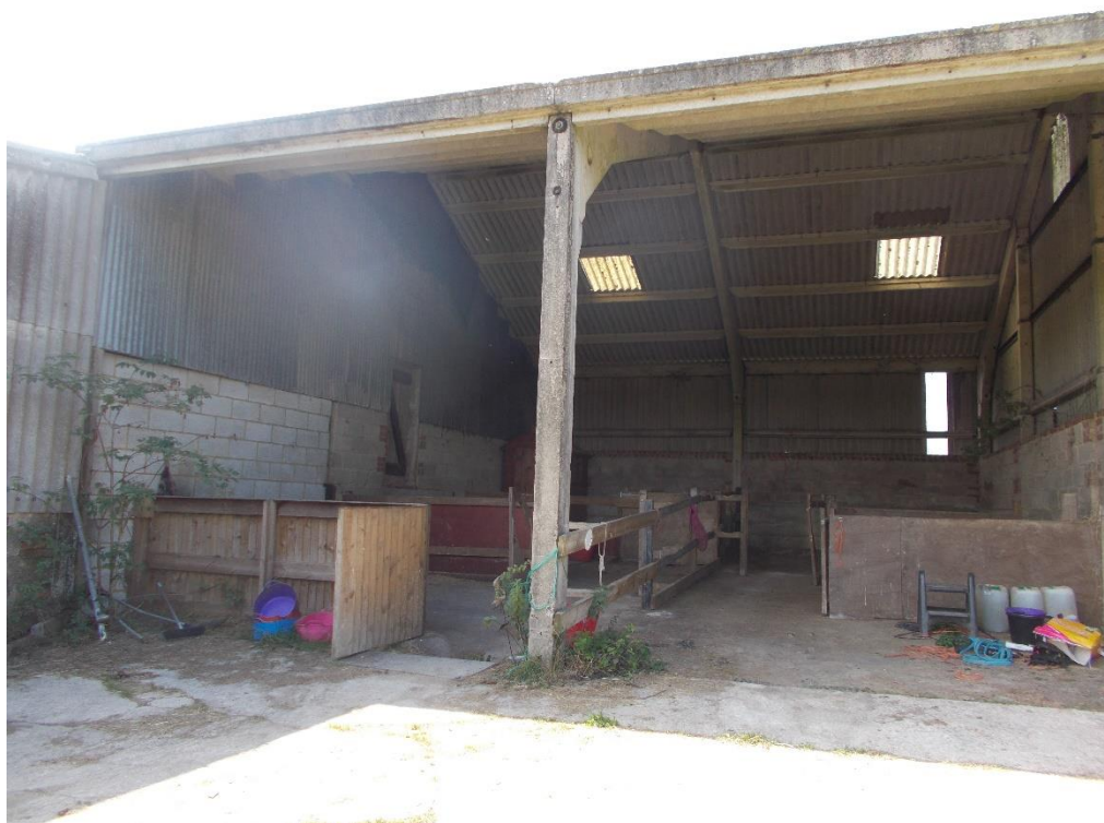
Photo 5: Loose boxes in rear extension.
