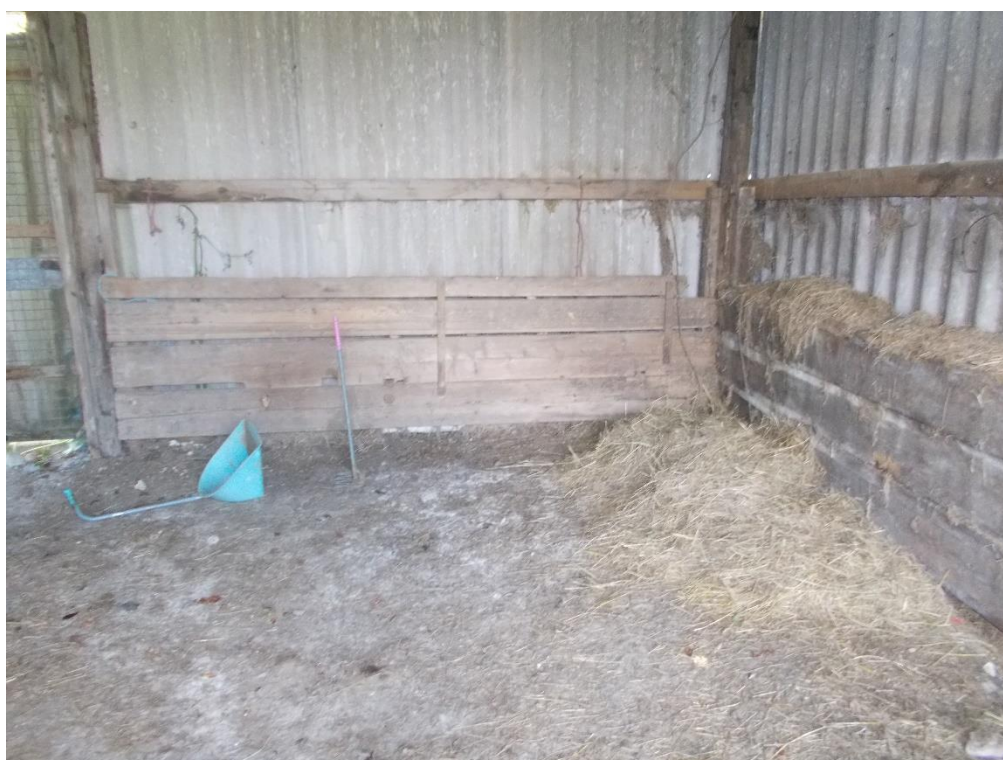
Photo 6: Smaller rear extension loose box.
