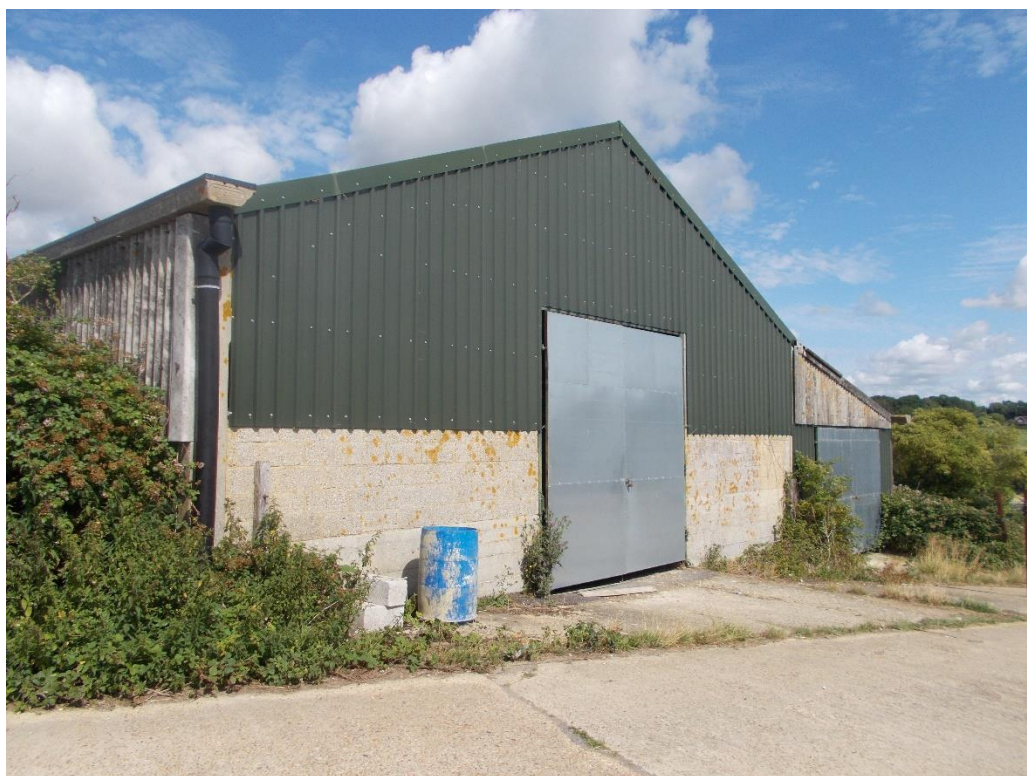
Photo 1: Front view of the barn and side extension.
