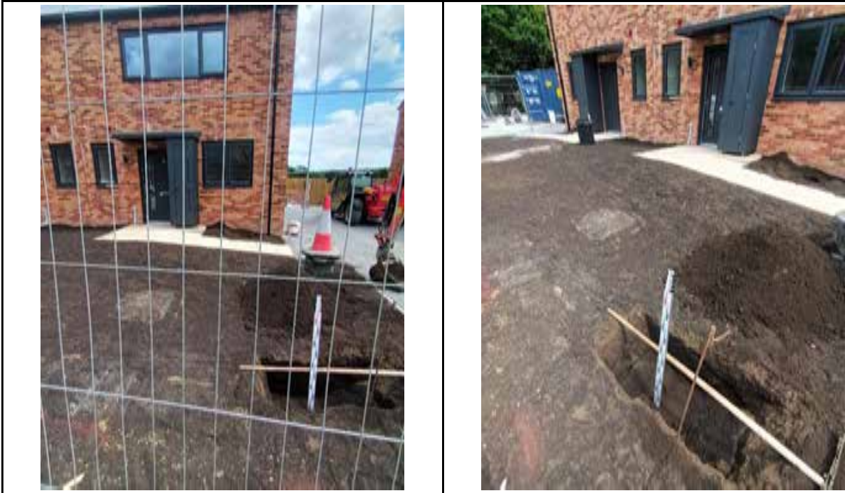
Contractor Photograph: Tree Pit – Front Garden No. 18
