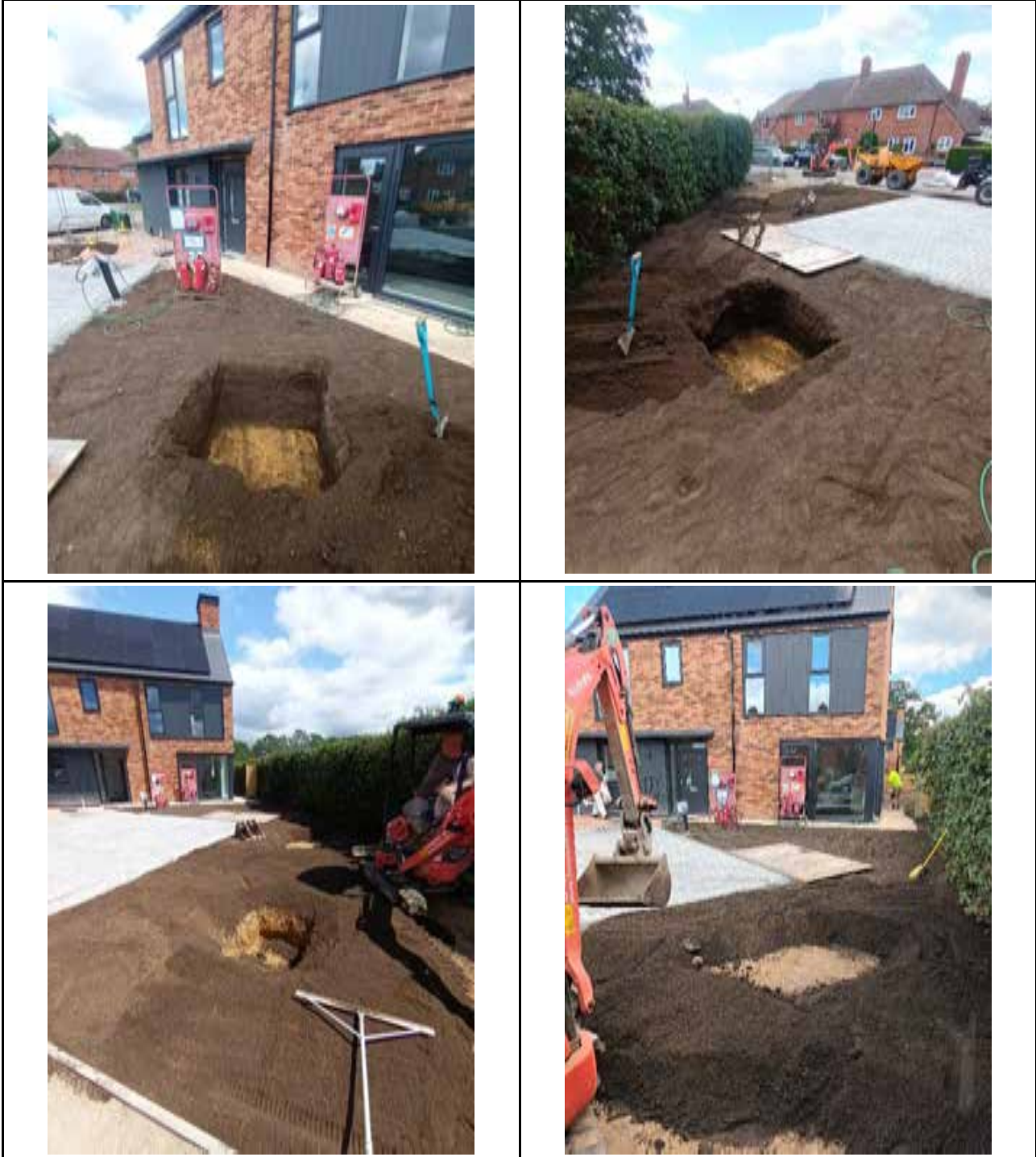
Contractor Photograph: Landscaped Area to the Front of No. 22
