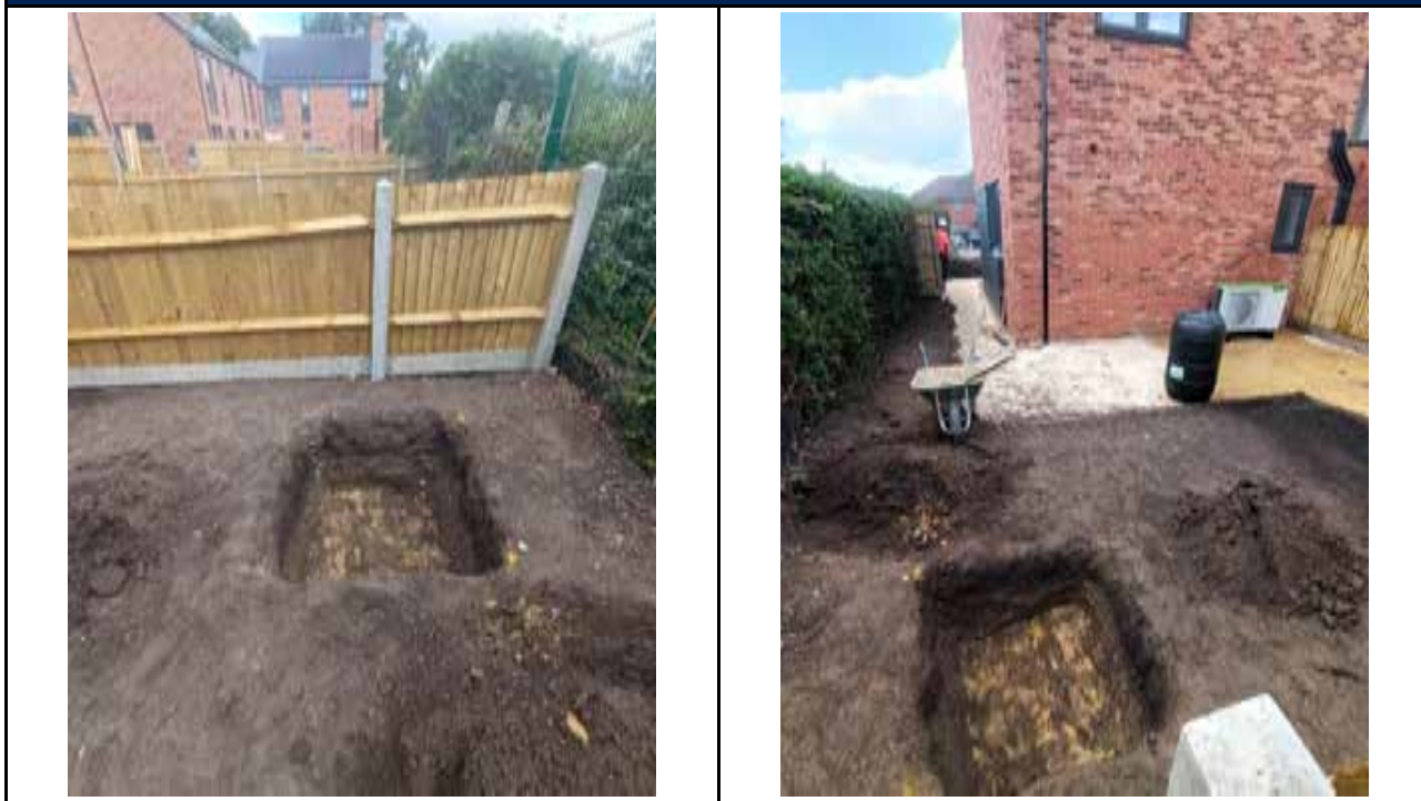
Contractor Photograph: Landscaped Area to the Front of No. 22
