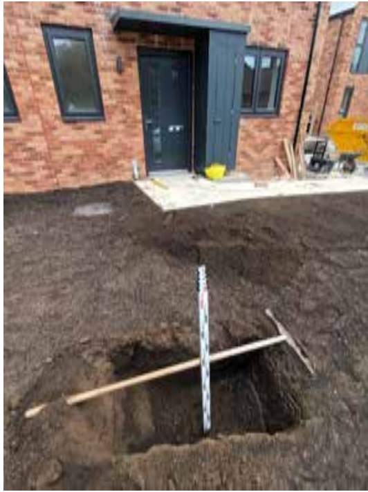
Contractor Photograph: Tree Pit – Front Garden No. 20
