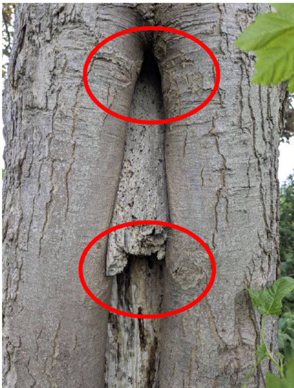
Figure 3. View of the tear out present on T28 with 2 PRF-Is identified (taken May 2025).
